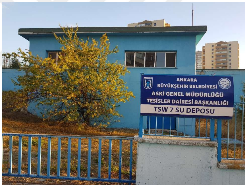
Figure 2.5 A water tank in Yaşamkent district.
