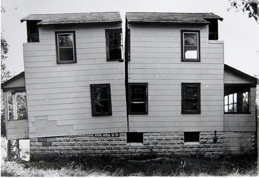
Resim 20. Gordon Matta- Clark, Ayırma , ( Splitting , 1974), New Jersey
