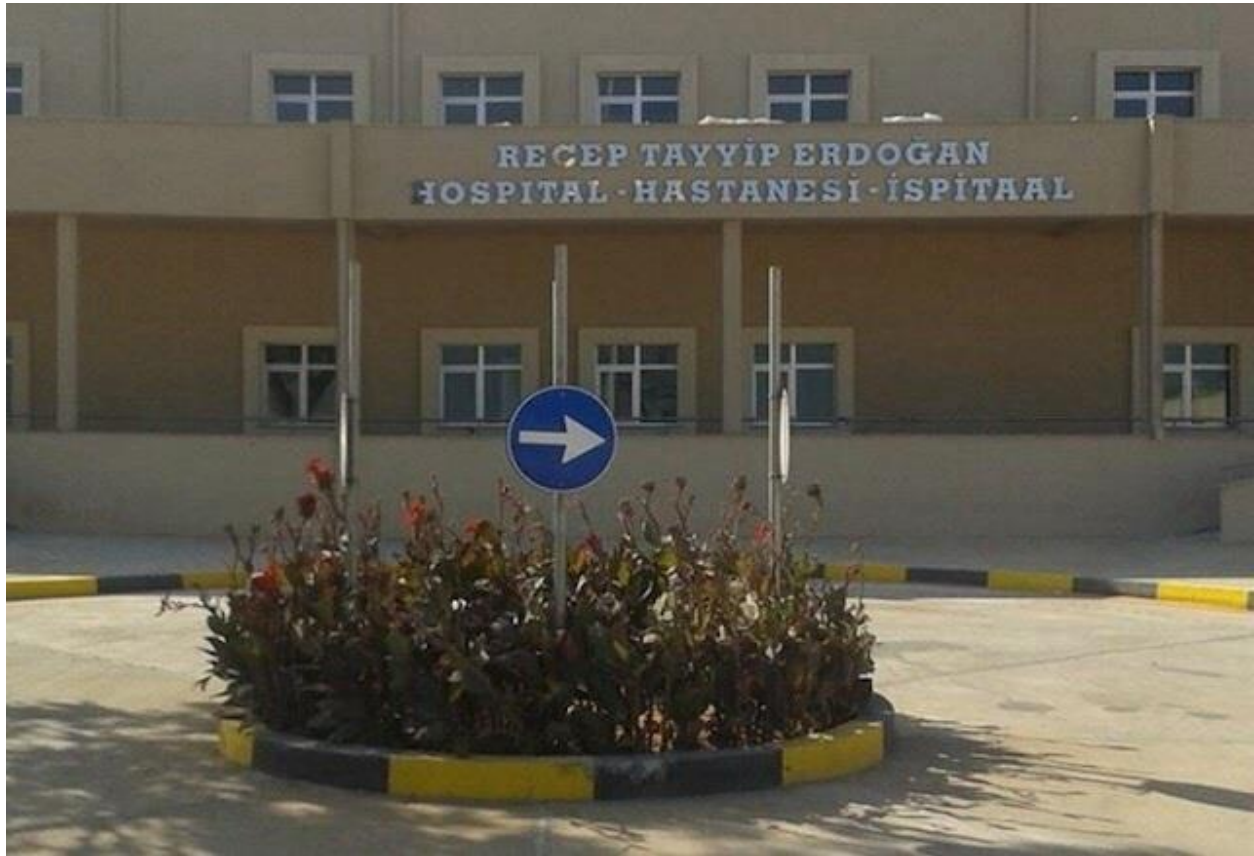
Figure 4.1: A section of the Recep Tayyip Erdogan Hospital (formerly known as Digfer Hospital)
