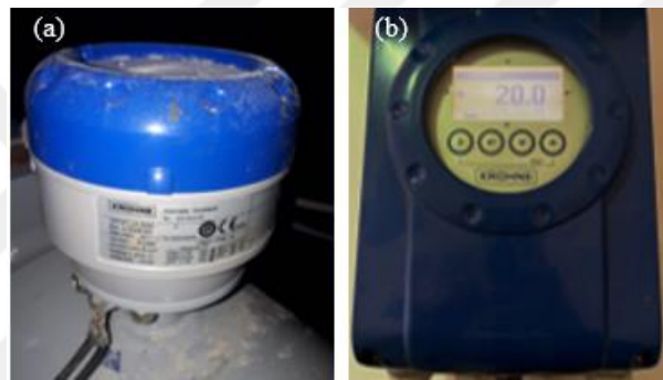
Figure 3.13: (a) and (b) Electromagnetic flowmeter
