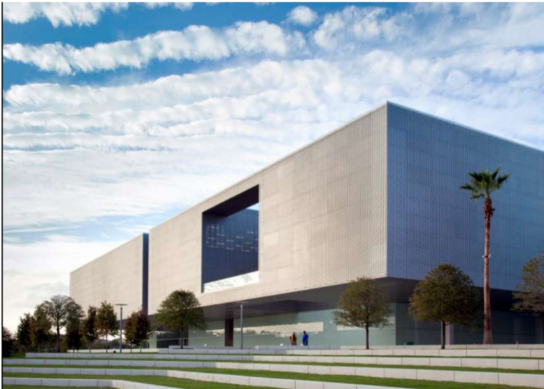
(Figure 3.1) Entrance Of The Tampa Museum
