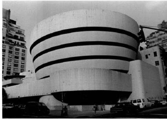
VIEW FROM SOUTHWEST
