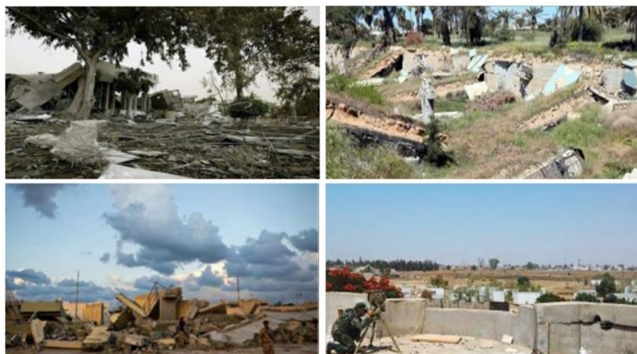
Figure 35: The Demolished Army Campos in Tripoli
