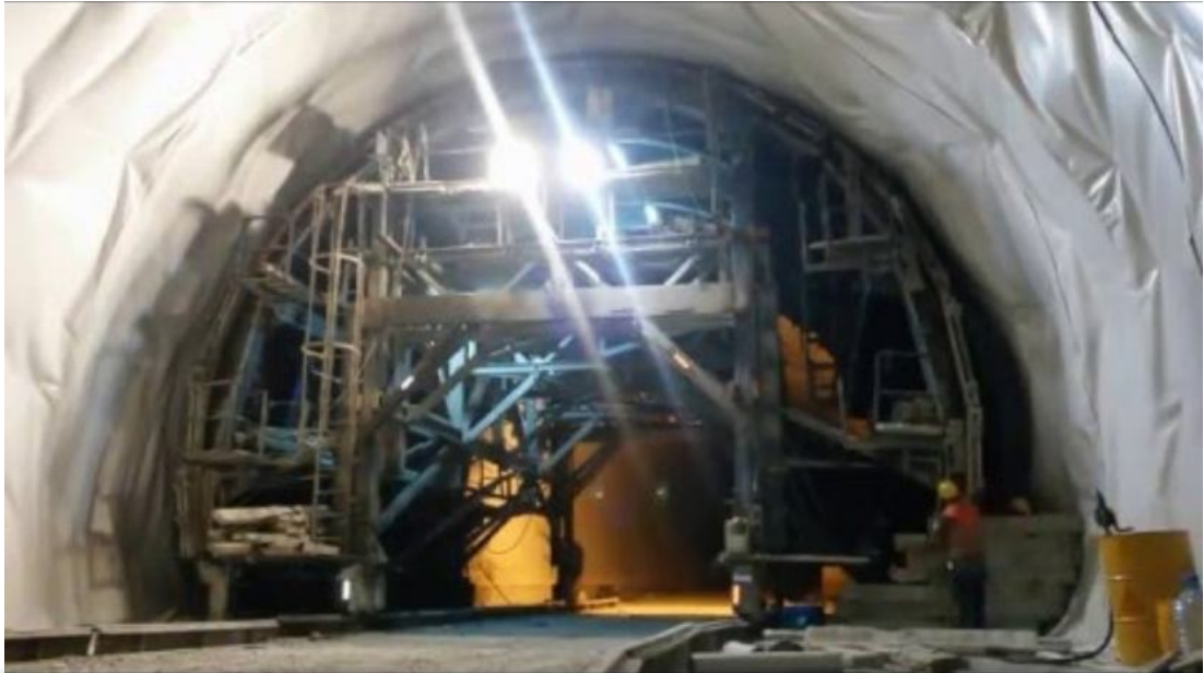
Figure 2.12 In tunnel mold Works [11].
