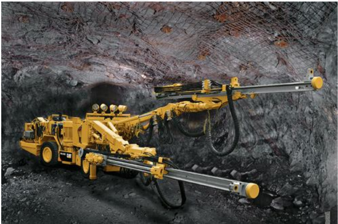
Figure 2.9 Drilling holes for insertion of explosives [11].
