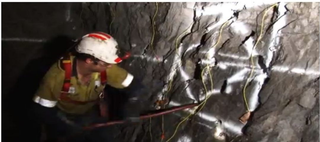
Figure 2.11 Installation of explosives in the tunnel mirror [11].
