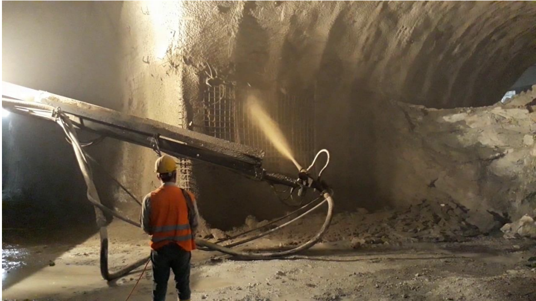
Figure 2.10 In tunnel scotcrete process [11].
