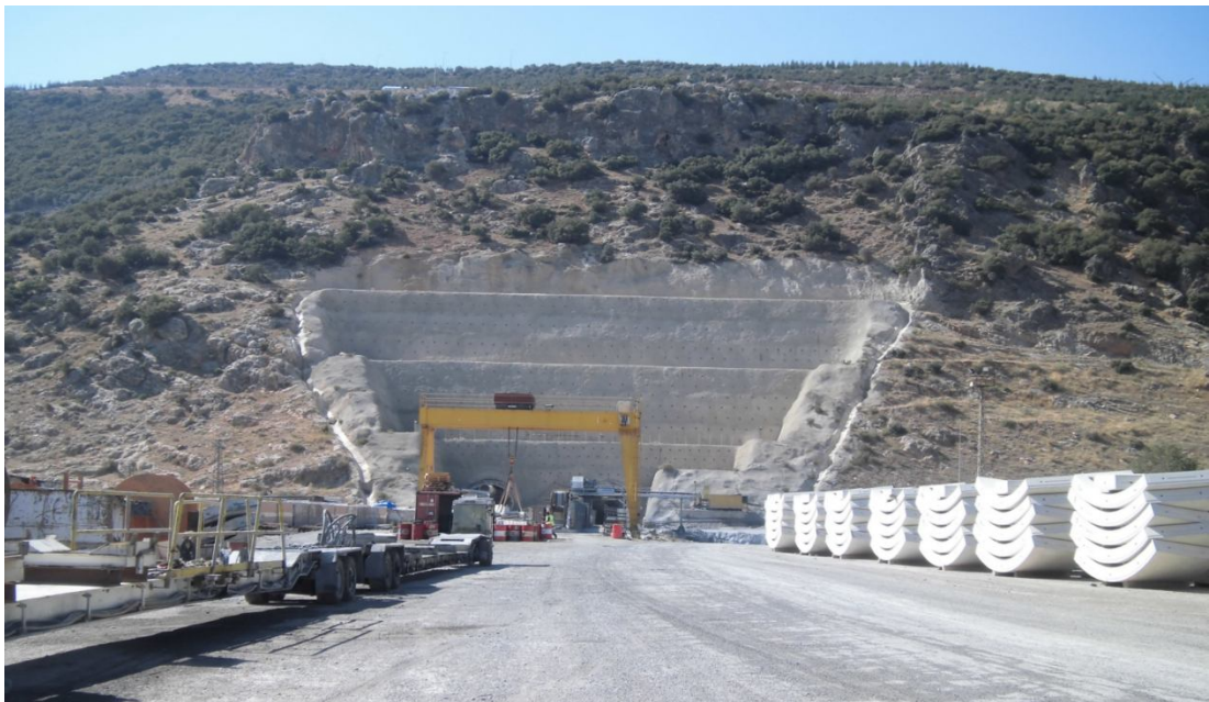
Figure 2.1 Bahçe-Nurdağı tunnel overview (By Musa BUDAK).
