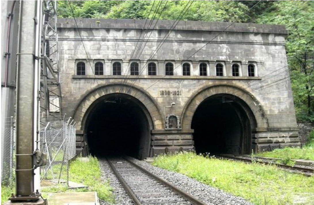
Figure 1.4 Simplon Tunnel (By Eugenio Merzagora).
