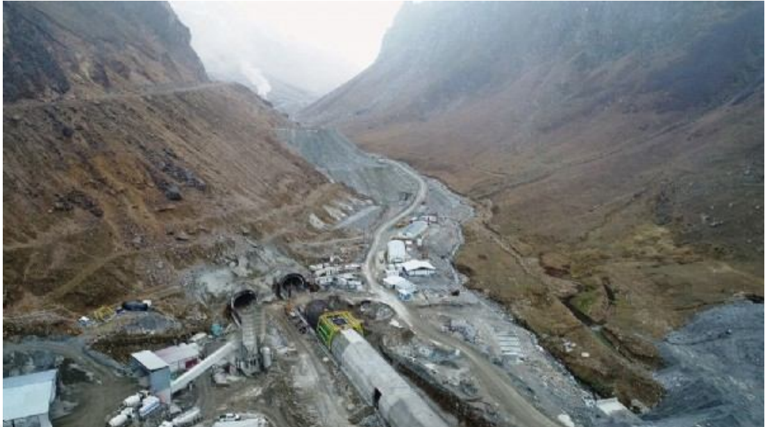
Figure 2.8 Tunnel construction site [11].
