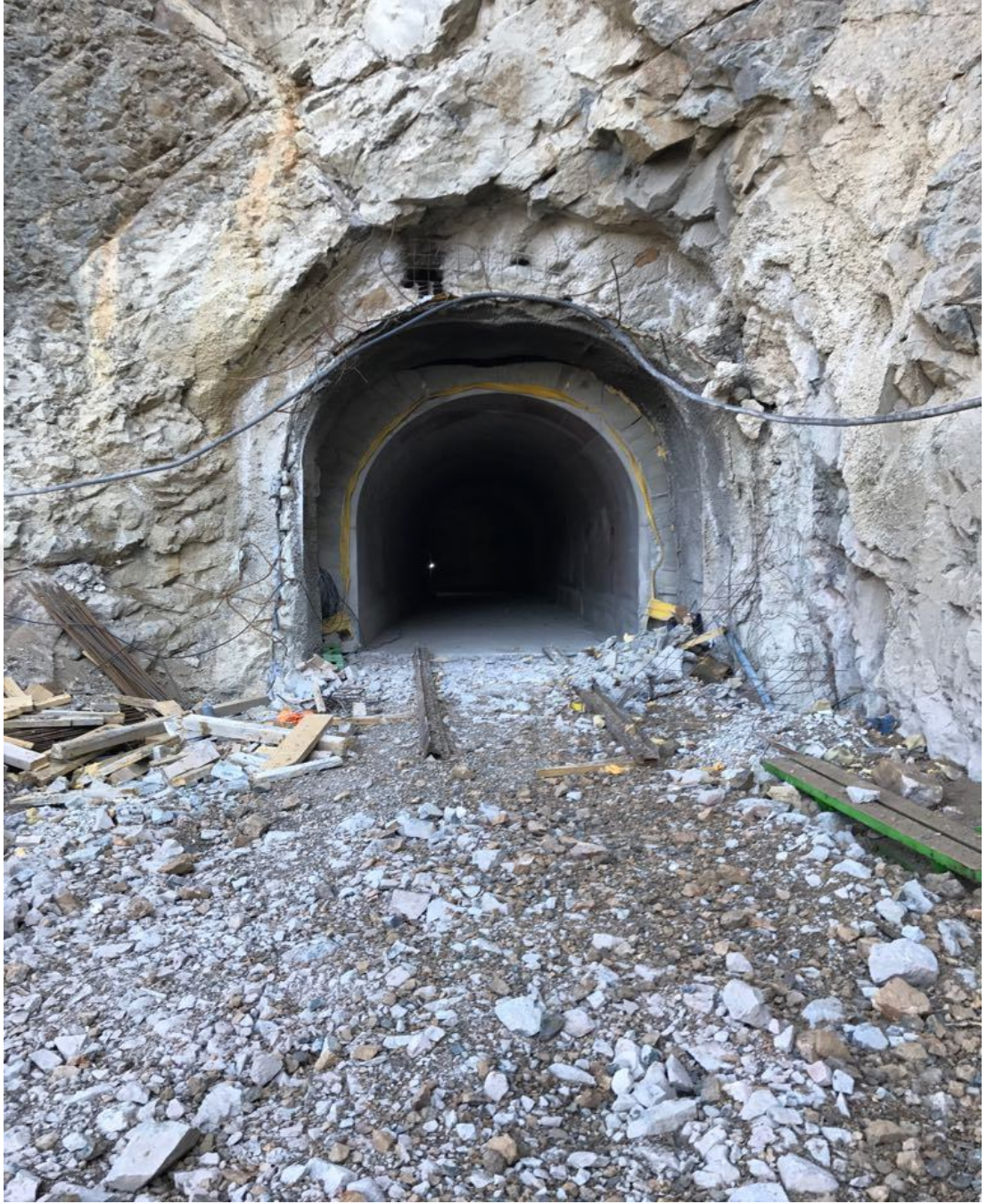
Figure 2.2 Artvin - Çoruh hydroelectric power plant transmission tunnel (By haldizinsaat.com.tr ).
