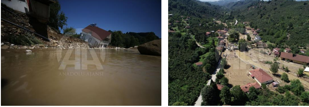
Figure 4. 5: The result and effect of 17-18 July 2019 flooding and landslide in Düzce Province, (Anadolu Agency, Url-5).
