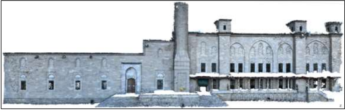
Figure 3.3: A 2,267,690 Point Cloud Model of the SW Facade, Captured from Agisoft Metashape.
