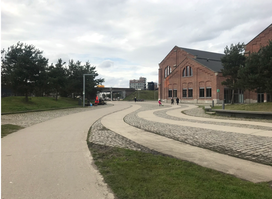
Figure 3.20 : Photo of the project.
