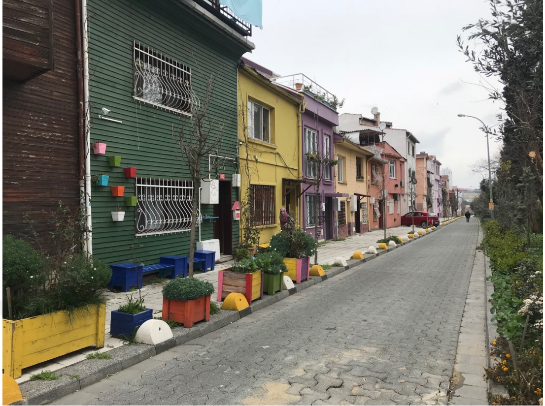
Figure 3.7 : Street renovations in the Yeldeğirmeni neighborhood.
