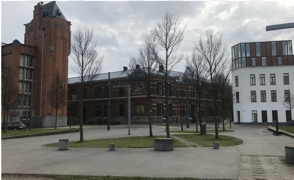
Figure 3.16 : Photo of the project.
