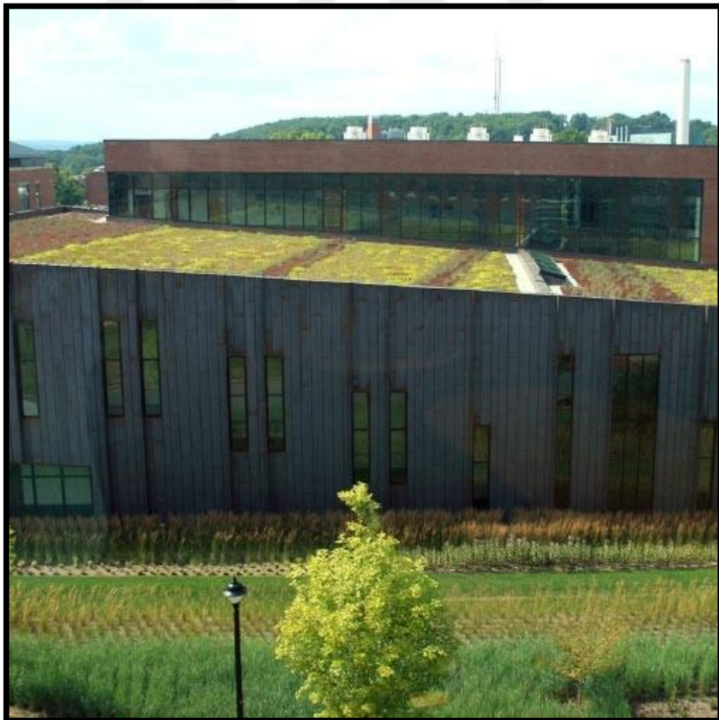
Figure 3.2. Green roofs in Connecticut University.
