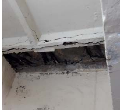
Figure B.45: Gnd-N/14 – Ticketing Booth – Deterioration (2016) Discoloration of paint on the western wall and the ceiling (left) Concrete chunk fallen off near the southern wall (right)
