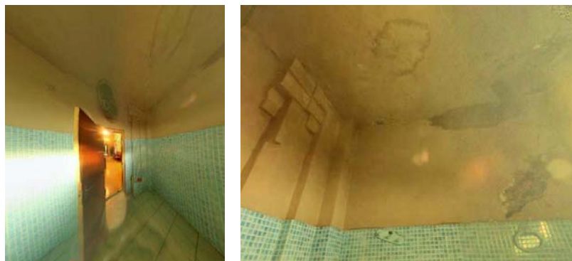
Figure B.75: Gnd-W/11 – Toilet for the Conference Room (2015) Looking North-East (left) Flaking of paint and efflorescence on eastern wall as well as discoloration on the ceiling due to dampness (right)
