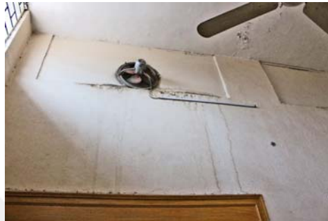
Figure B.104: Fst-E/13 – Freedom Movement Gallery – Deterioration (2015) Drip marks on the northern wall
