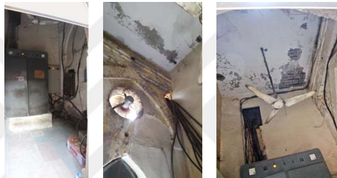
Figure B.65: Gnd-S/13 – Electric Control Room (2016) Looking North (left) Flaking of paint observed on the Southern wall and on the ceiling (center) Looking North-East flaking of paint observed on the Eastern wall as well as detachment of concrete from ceiling (right)
