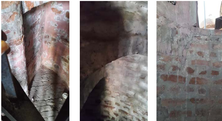
Figure B.42: Gnd-N/11 – North Western Stairwell (2016) Powdering of brick and mortar on the central column and the periphery wall (left) Steps supported on brickwork arches (center) Crack towards the North, halfway to the first floor (right)
