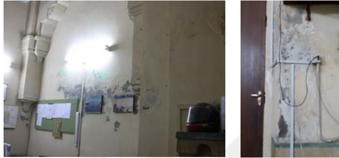
Figure B.37: Gnd-N/04 – Office of Chief Security Officer – Deterioration (2015) Flaking of paint on the Western wall (left) Flaking of paint and discoloration Northern wall (right)
