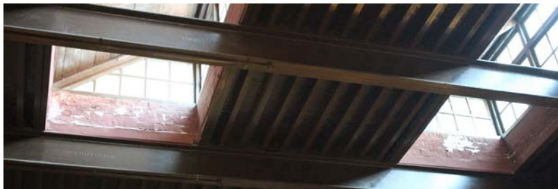
Figure B.12: Gnd-E/02 – Gandhara Gallery – Deterioration (2016) Efflorescence on brick masonry supporting skylight
