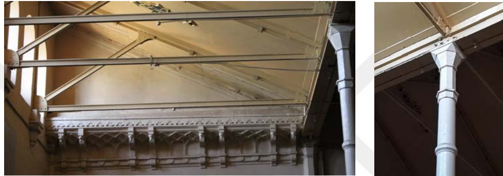
Figure B.9: Gnd-E/01 – Islamic Arts Gallery – Structural Components (2016) Saw Tooth Trusses built with railway girders (left) Cast Iron Columns supporting compound girders which in turn support the trusses (right)
