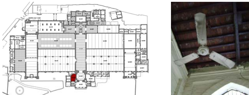
Figure 2.53: Lahore Museum key plans showing location of T-Iron Brick Roof supported on I-Beams in space Gnd-N/04 (left) Looking South at T-Iron Brick Roof in Space Gnd-N/04 (right)
