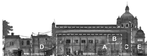
Figure 2.28: Lahore Museum – Eastern Façade (2016) Orthographic projection from laser scan point-clouds A: Laboratory, B/C/D: Galleries, E: Frontispiece Source: Sami (2017, p. 108)
