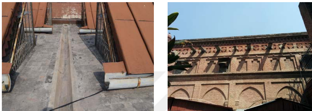
Figure 2.79: Sloping roofs draining into gutter which discharge onto flat roof (left) Roof draining directly onto Southern Façade through scuppers (right)
