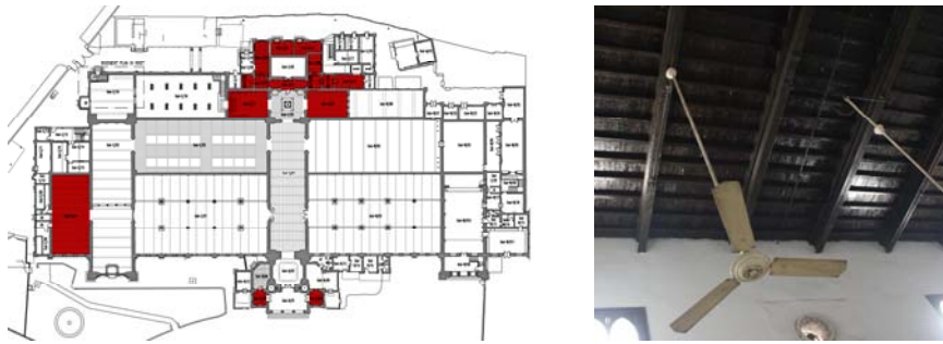
Figure 2.50: Lahore Museum key plans showing locations of I-Beam supporting Wooden Flat Roofs (left) Looking South at Wooden Flat Roof supported on I-Beams in Space Gnd-W/07 (right)
