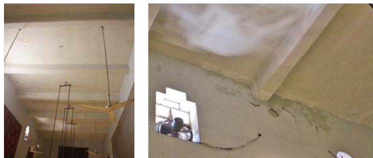
Figure B.34: Gnd-W/08 – Swat Gallery (II) – Deterioration (2016) Discoloration due to dampness on the ceiling around the electric points (left) Flaking of paint on the Southern wall close to the ceiling
