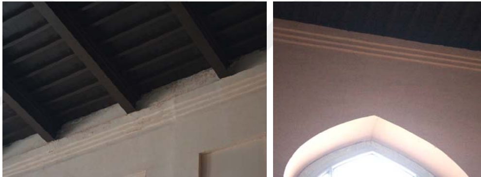
Figure B.16: Gnd-E/04 – Pre and Proto Historic Gallery – Deterioration (2016) Discoloration and flaking of paint near the ceiling on the Eastern wall (left) Vertical crack passing through the central window on the Northern wall (right)
