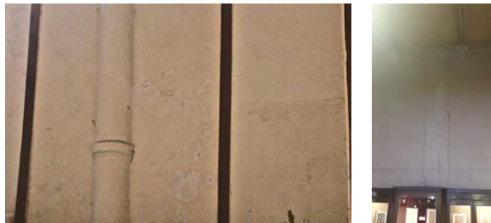
Figure B.25: Gnd-W/01 – General Gallery (2016) Flaking of paint and discoloration due to dampness on the Northern wall (left) Drip marks flowing down from the ceiling on the Southern Wall (right)
