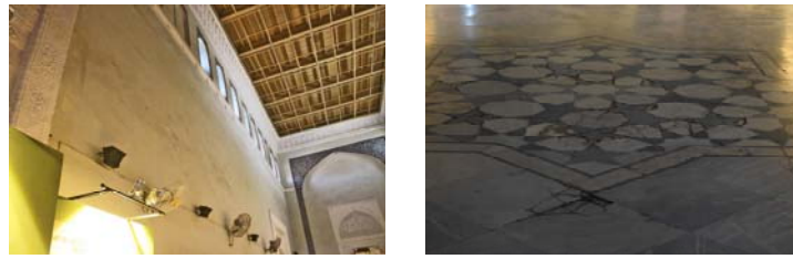
Figure B.6: Gnd-C/01 – Miniature Painting Gallery – Deterioration (2017) Swelling of Plaster on the Eastern Wall (left) Marble floor pattern cracked (right)
