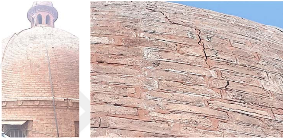
Figure 2.77: The meridional cracks observed on the Main Dome (left) Close-up showing the crack breaking brick unit (right)
