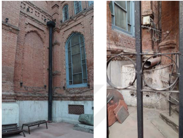
Figure 2.74: Two downspouts one at the eastern end (left) and the other at the western end (right) of the wall Gnd-E/01-N-W. Concrete walkway can also be seen in the images
