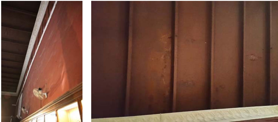
Figure B.14: Gnd-E/03 – Hindu and Buddhist Gallery (2017) Plaster swelling on Eastern wall (left) Discoloration due to dampness on roof (right)
