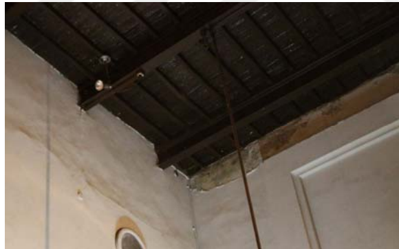
Figure B.21: Gnd-E/17 – Jain Gallery (II) – Deterioration (2016) Swelling of plaster on the South wall while flaking of paint on the Western wall
