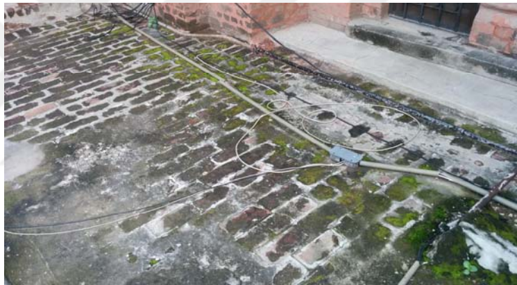
Figure B.86: Fst-N/03 – Terrace – Deterioration (2015) Microbiological growth on the floor
