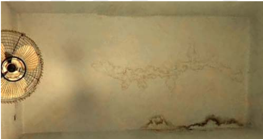
Figure B.18: Gnd-E/05 – Men's Toilet – Deterioration (2015) Discoloration of paint due to dampness on the ceiling
