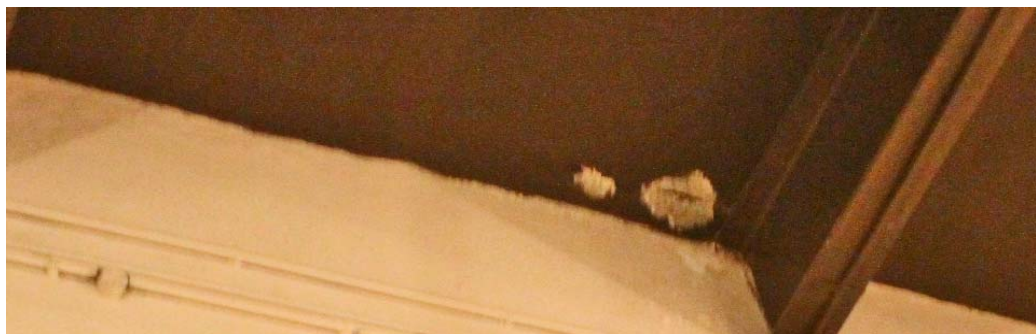
Figure B.27: Gnd-W/02 – Contemporary Painting Gallery (2016) Detached chunk of concrete near the Southern wall
