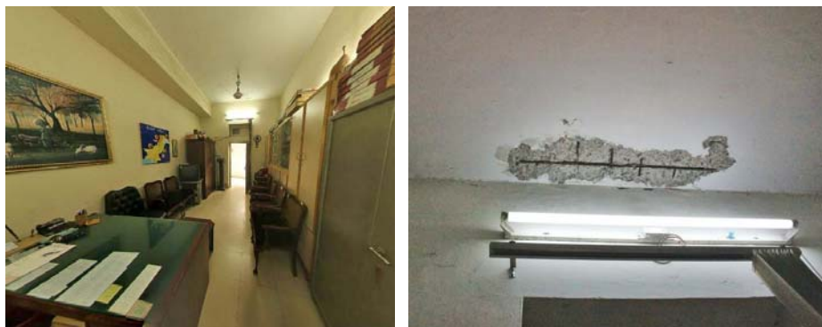
Figure B.70: Gnd-S/19 – Office (2015) Looking South (left) Detachment of concrete from ceiling at the Southern end of the room (right)
