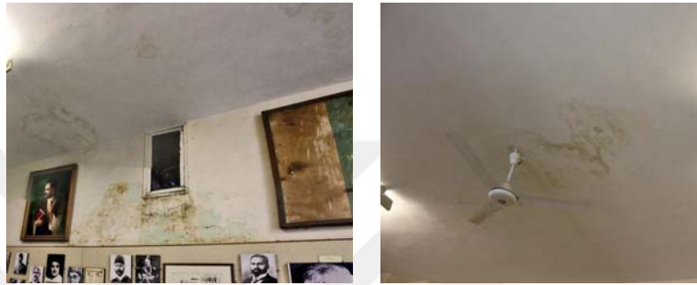
Figure B.106: Fst-E/15 – Freedom Movement Gallery (II) – Deterioration (2016) Flaking of paint and drip marks on the Eastern wall (left) Drip marks and discoloration of paint on the ceiling (right)
