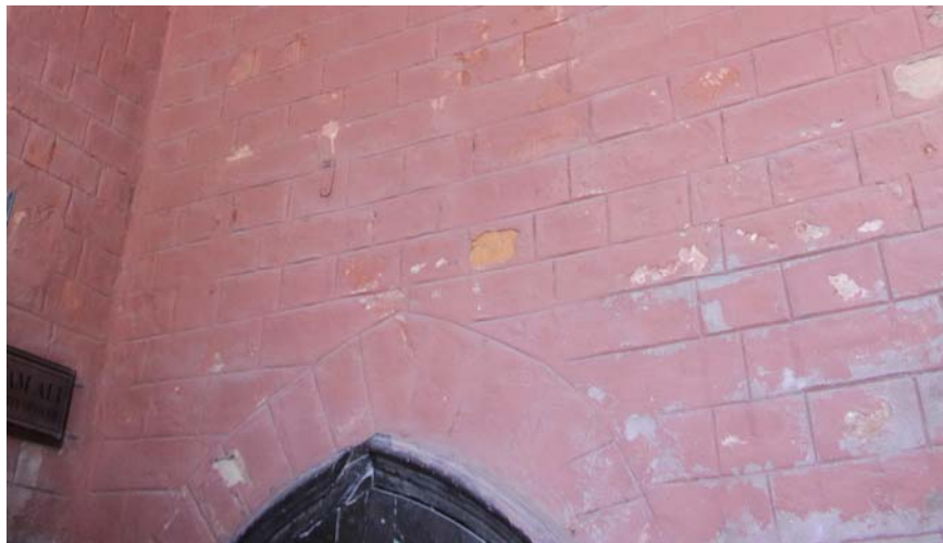
Figure B.2: Gnd-N/01 – Entrance Portico (2017) Flaking of red tinted cement layer and powdering of brick
