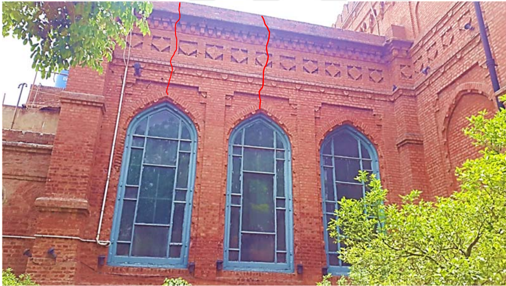
Figure 3.32: Vertical Cracks (S1) Through the Central and Eastern Arch of Gnd-E/04-N-W (2017)
