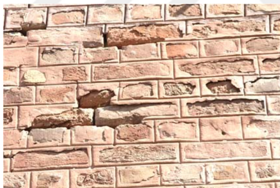
Figure 2.81: Powdering of Brick / Detachment of Pointing on the exterior wall of Fst-W/01 (2017)
