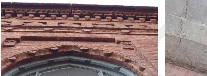
Figure 2.71: Vertical Crack going through Central Arch of Gnd-E/04-N-W (2015) Crack starts from the parapet (left) and reaches till the base of the wall (right)
