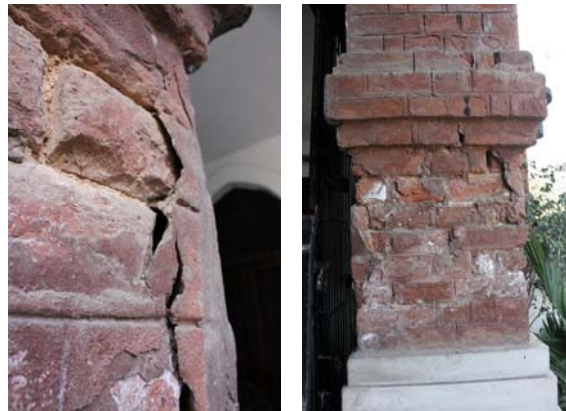
Figure B.72: Gnd-W/09 – Entrance Lobby to the Auditorium and Library – Deteriorations (2016) Efflorescence as well as a powdering and detachment of bricks
