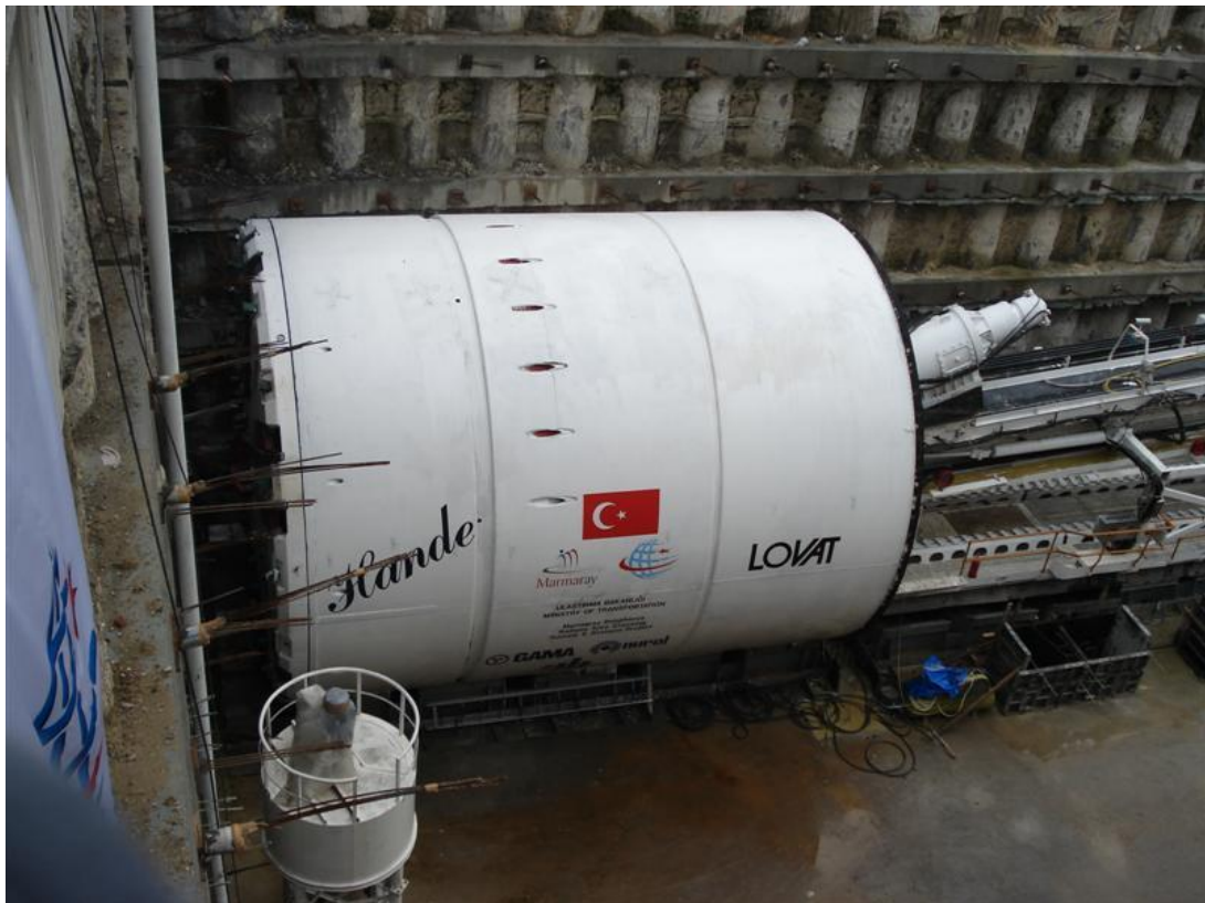
Figure 3.5: Tunnel Boring Machine – TBM-1
