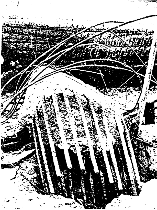
PHOTO B.1 Failure of a column due to insufficient anchorage. (San Fernando Earthquake of 1971), ATC (1979).
