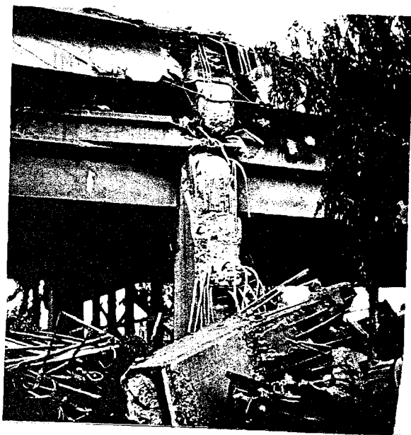
PHOTO B.5 Cypress Avenue (I-880) double deck crossing. (Loma Prieta Earthquake of October 17, 1989), Time (October 30, 1989).
