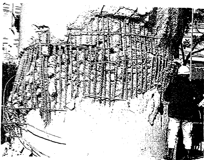
PHOTO B.12 Close view of mid-height pier damage on Hanshin Expressway.
