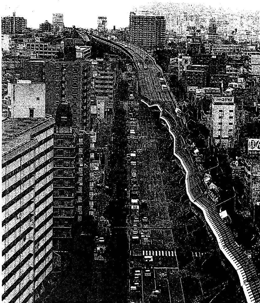
PHOTO B.7 Collapse of Hanshin Expressway. (Kobe Earthquake of January 17, 1995), (Aydinoğlu N., 1995).
