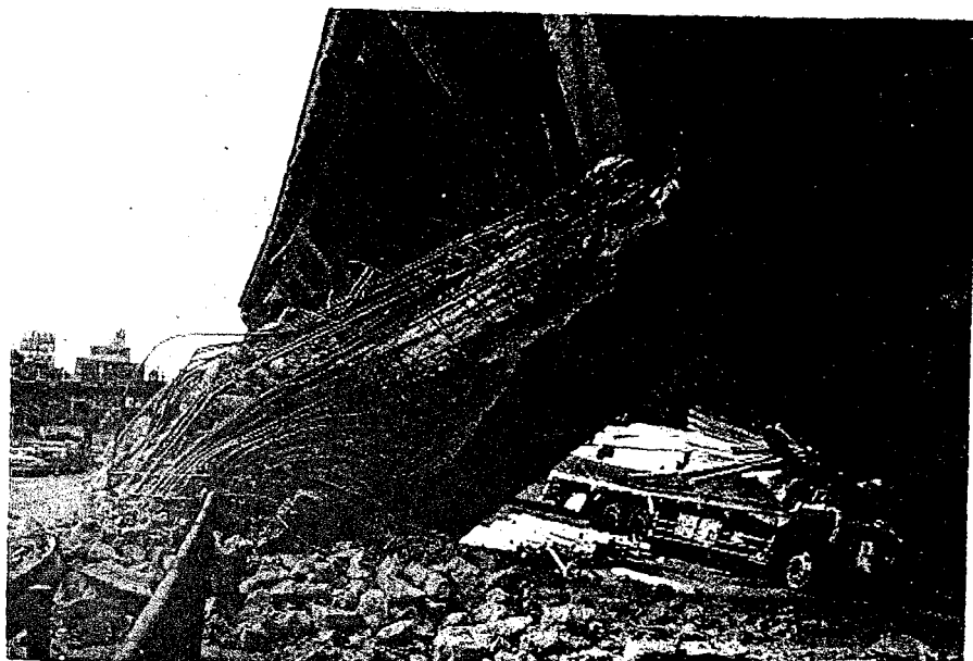
PHOTO B.9 Close view of a broken pier of Hanshin Expressway. (Kobe Earthquake of January 17, 1995), (Aydinoğlu N., 1995).
