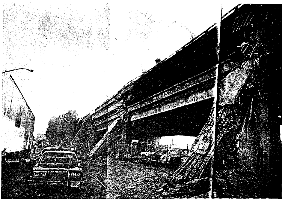
PHOTO B.6 Cypress Avenue (I-880) double deck crossing. (Loma Prieta Earthquake of October 17, 1989), Time (October 30, 1989).
