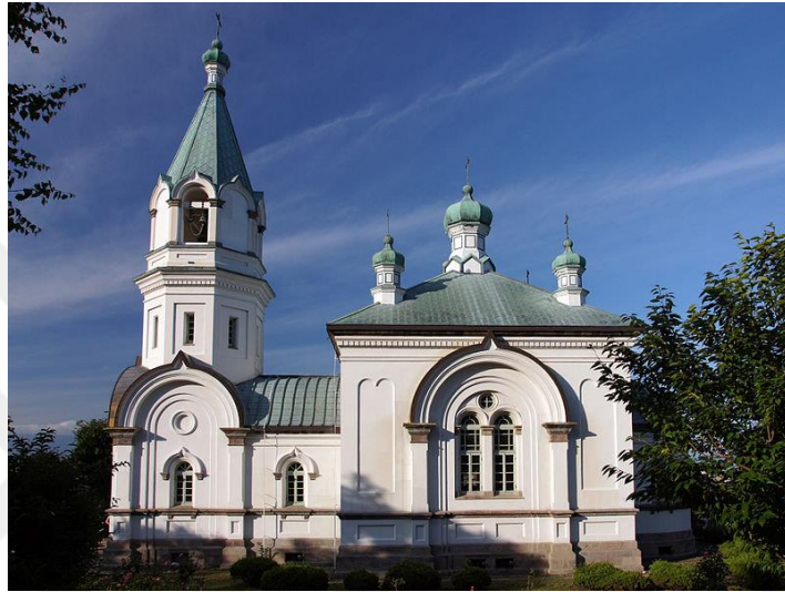
Figure 3. 1: Holy Resurrection Orthodox Church of Hakodate,Hokkaido,Japan, current site dated from 1916. [URL 8]
