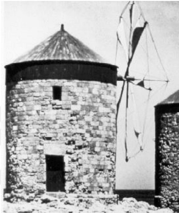
Figure 2.2. An Early European Horizontal Axis Windmill [24].
