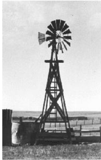
Figure 2.3. A Steel Blade Water Pumping Windmill [25].
