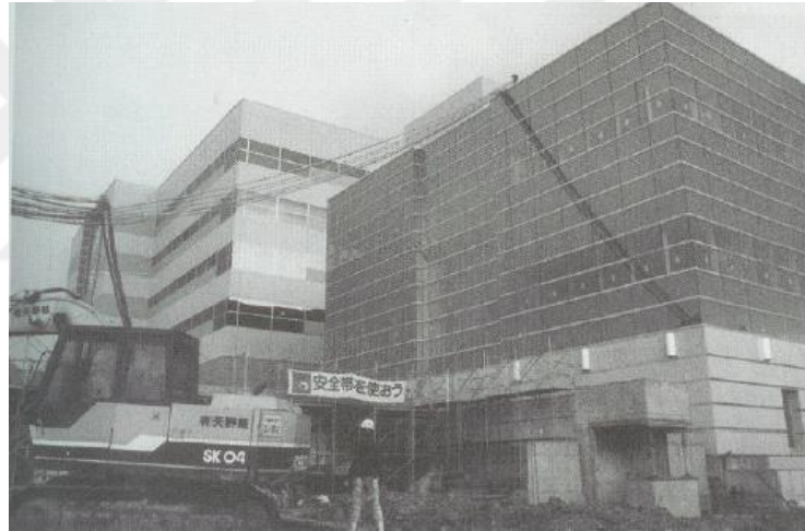
Şekil 1.14 Technical Research Institute of the Matsumura-Gumi Construction Company binası (Urgu, 2006)
