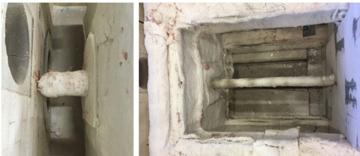
Figure 3.46. Insulated socket head (left-hand side) and insulation of the specimen S5 with ceramic fiber blanket (right-hand side).
