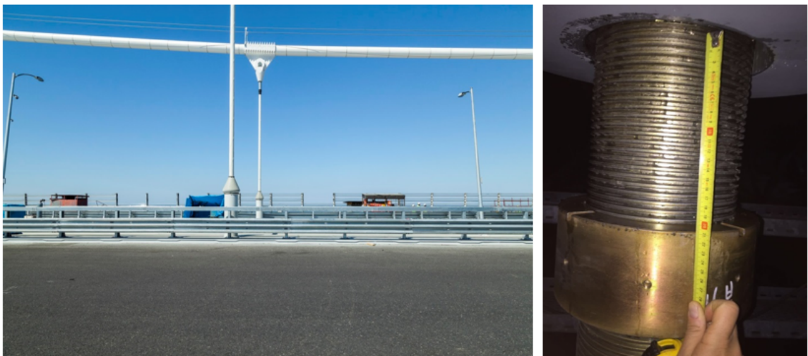
Figure 1.3. Typical suspender system components; main cable, cable band, suspender cable (left-hand side), End Anchor of cable; socket and nut (right-hand side).
