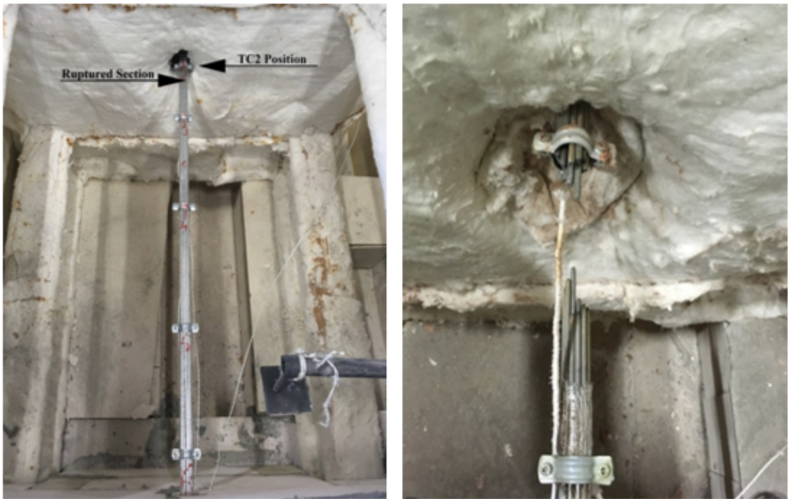
Figure 4.21. TC2 position prior to Test 4 and front view of ruptured section.
