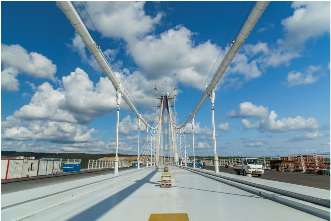
Figure 1.2. Passing through a vehicle nearby the suspender cable.
