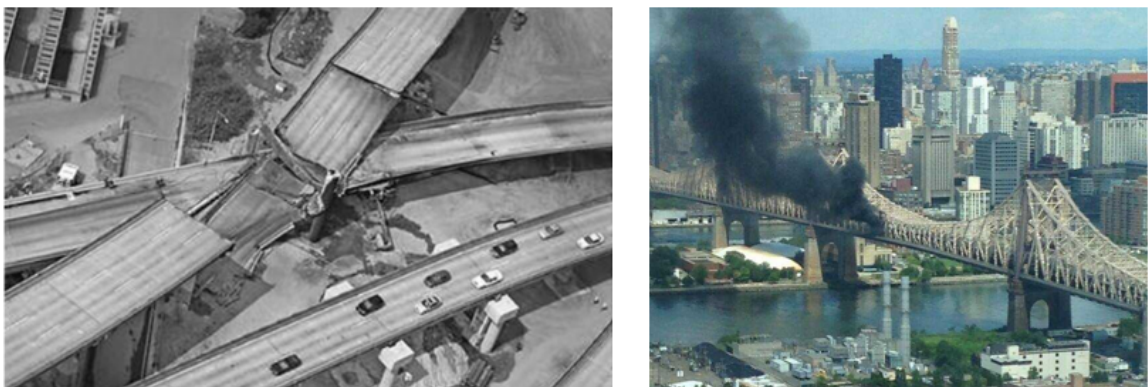
Figure 2.16. Oakland Highway Bridge collapse, 2007 (left-hand side), Queensboro Bridge Fire hazard, 2013 (right-hand side).
