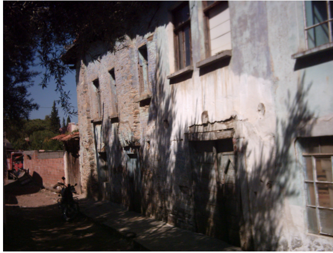
Figure 106, Case 19, Exterior view (Taşdöğen)
