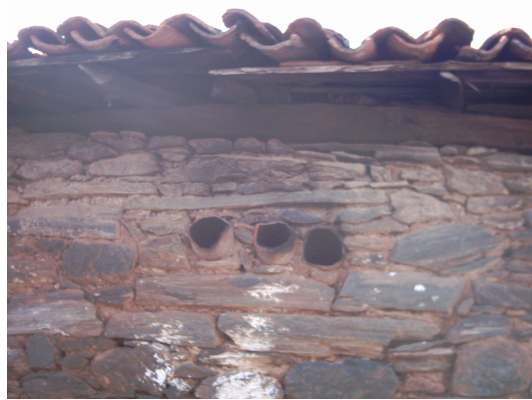
Figure 156, Chimney elements in the facade, an example from Karşıyaka (Taşdöğen)
