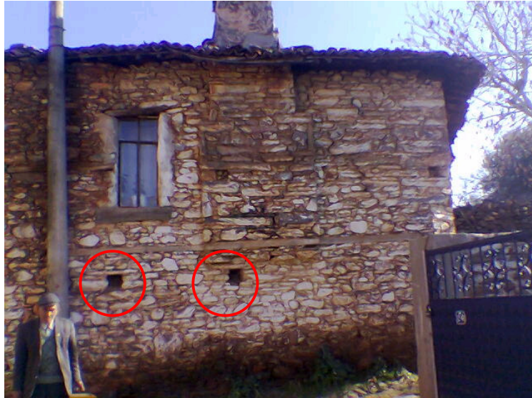
Figure 154, A dwelling in Hacı Arap Street, Karşıyaka, exterior wall with ventilation niches (Taşdöğen)
