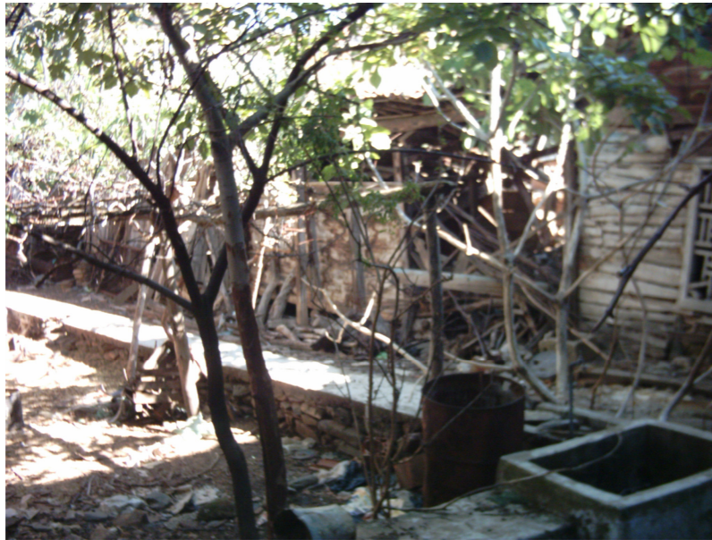
Figure 85, Case9, Footpath in the courtyard (Taşdöğen)
