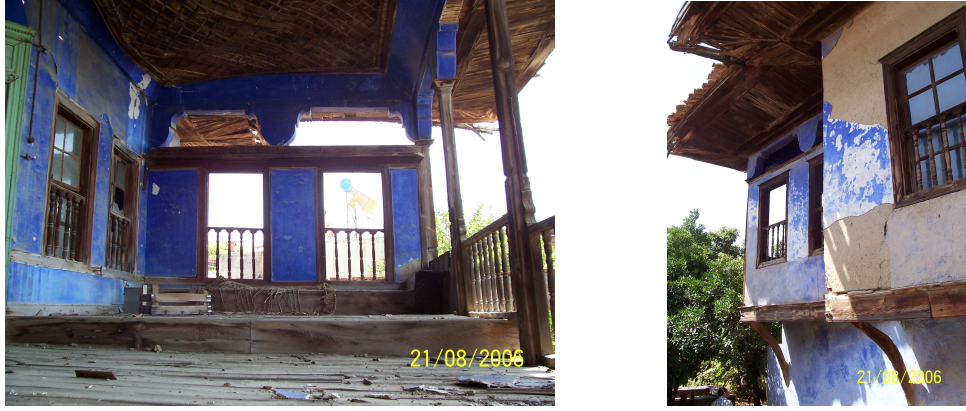
Figure 34, Hulusi Yalçın dwelling (Kuyucak), schematic plans of the house and views from hayat and eliboğründe (Taşdöğen)
