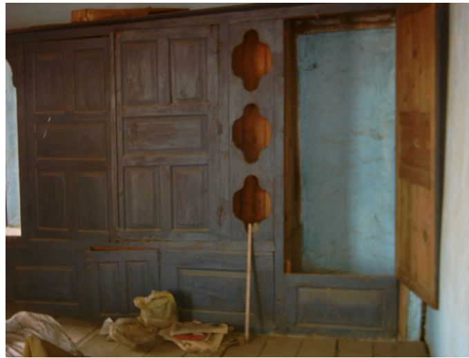
Figure 140, Cupboards in rooms (Taşdöğen)
