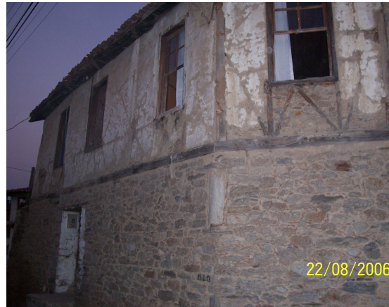
Figure 39, A traditional Bozdoğan dwelling with timber skeleton system (Taşdöğen)
