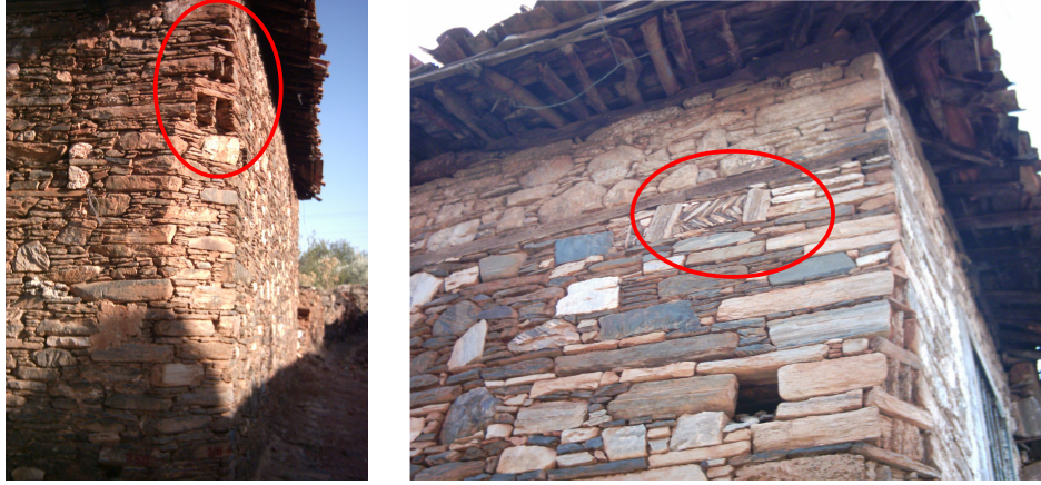
Figure 155, Corner details created with stone in Karşıyaka (Taşdöğen)
