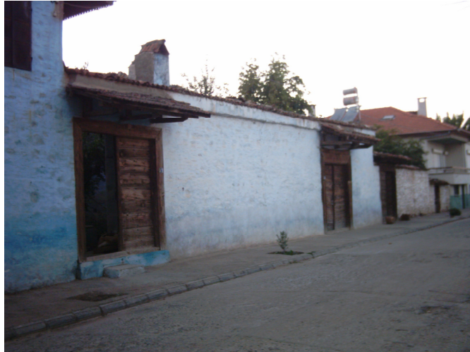
Figure 82, Case 8, Entrances of the two dwellings in the adjacent plots (Taşdöğen)
