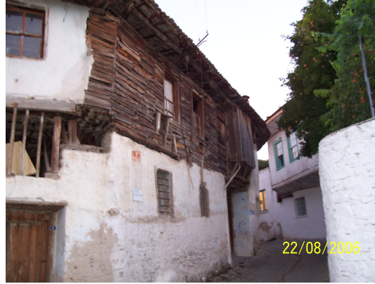
Figure 38, A traditional Bozdoğan dwelling with timber covering (Taşdöğen)
