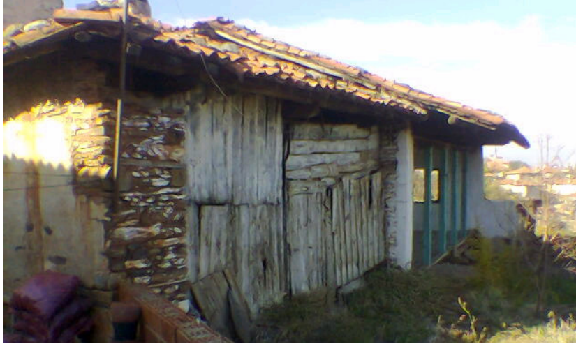
Figure 110, Case 23, View from courtyard (Taşdöğen)
