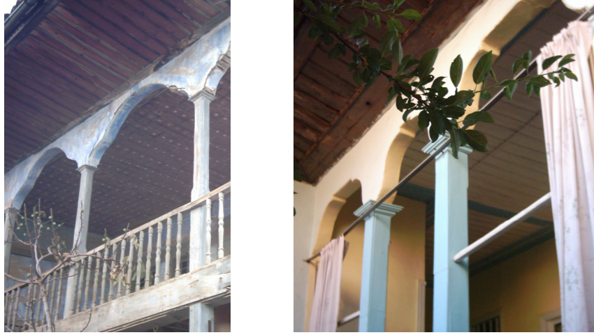
Figure 132, Timber colonnades with Bursa-type arches in hayats of a demolished dwelling and Case 1 (Taşdöğen)
