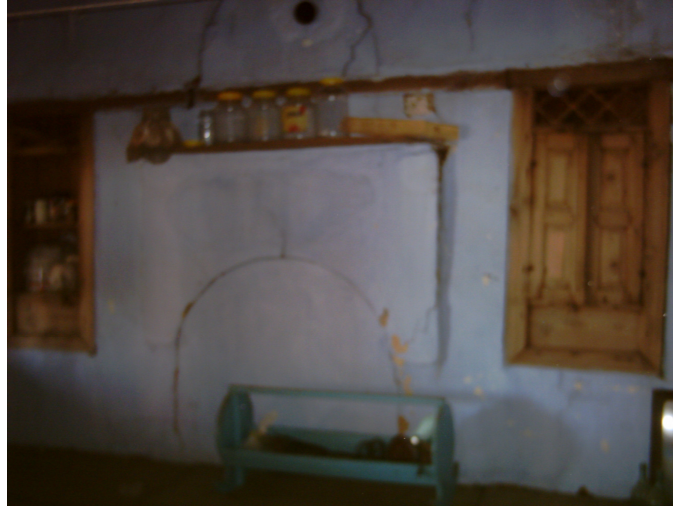
Figure 94, Case 11, Walled hearth (Taşdöğen)
