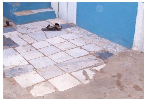
Figure 144, Case 1, Marble pavement (Taşdöğen)
