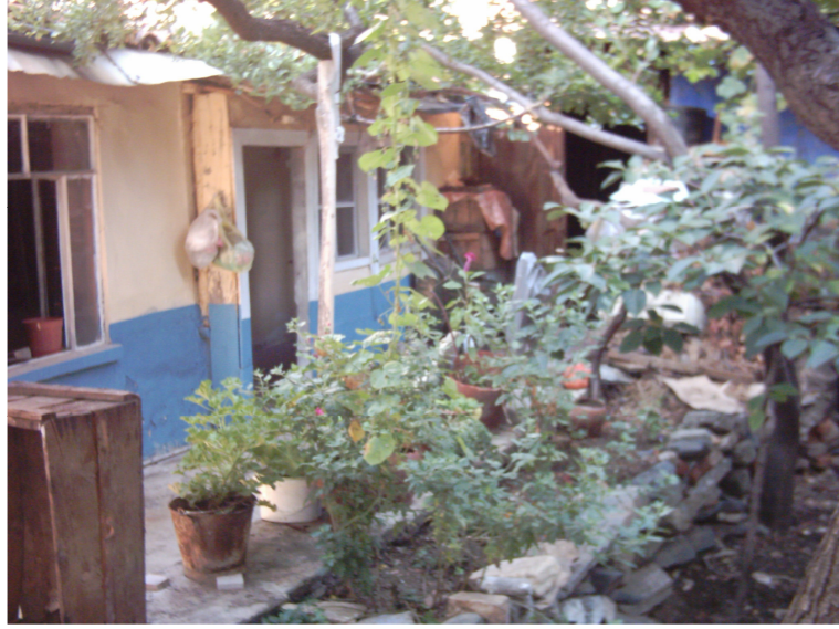
Figure 53, View of the services in the courtyard (Taşdöğen)
