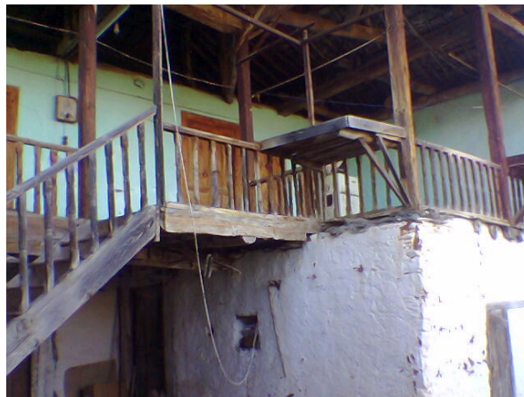
Figure 149, A dwelling in Hacı Arap Street, Karşıyaka; an example without ceiling in hayat (Taşdöğen)
