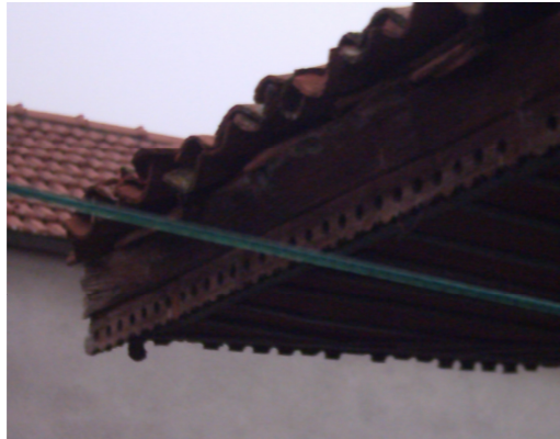
Figure 151, A type of eave (Taşdöğen)
