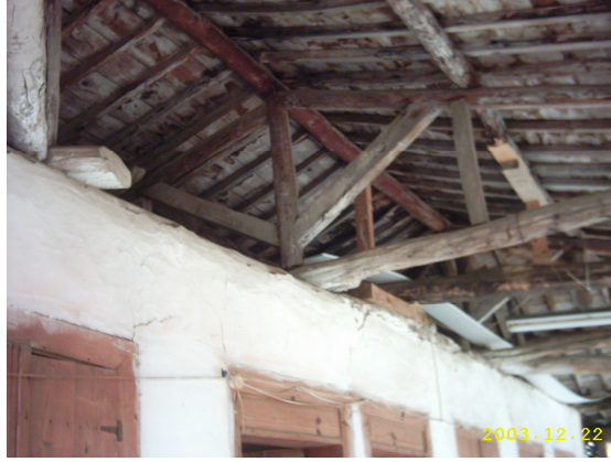
Figure 150, A plateau dwelling without a ceiling in hayat (Taşdöğen)
