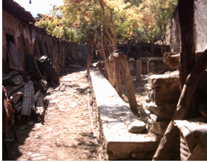
Figure 128, Case 9, footpath in the courtyard (Taşdöğen)
