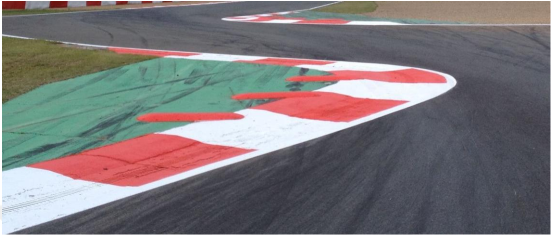
Figure 3.7 Kerbs on the road bend of the Circuit de Zolder (Personal archive, 2022)
