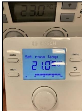
Figure 5.1 Operating with Bosch CR50 OpenTherm thermostat (Personnel Archive, 2023)
