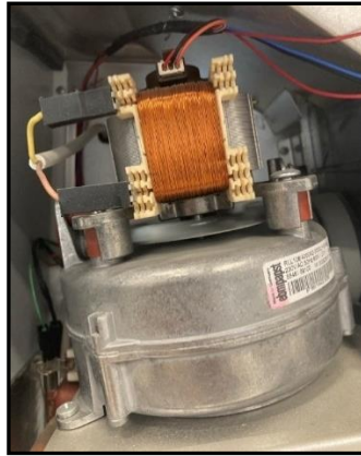
Figure 3.26 Bosch Condens 2000 W fan (Personnel Archive, 2023)
