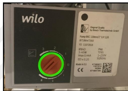
Figure 3.24 WILO RKC circulation pump (Personnel Archive, 2023)
