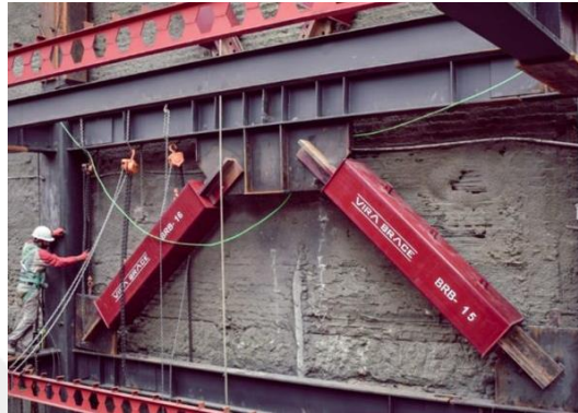
Figure 1.5: Buckling-restrained braces ( taken from Vira Brace Inc. )
