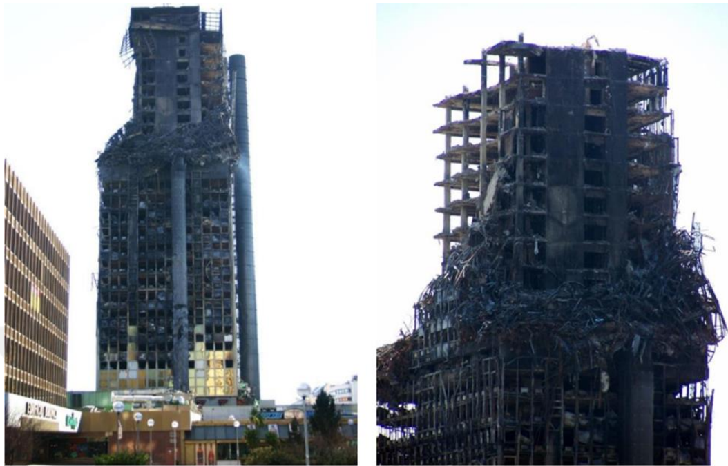
Figure 1.6. The Windsor Tower in Madrid after a 26-hour fire in 2005 (Ghali, et al., 2015).
