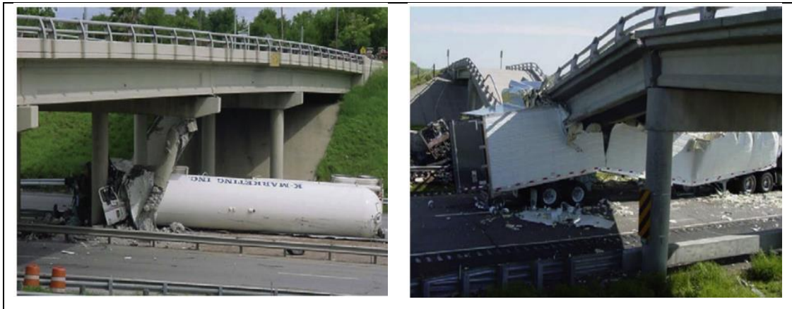
Figure 1.2. Failure of the bridge column as a result of a collision with a truck.
