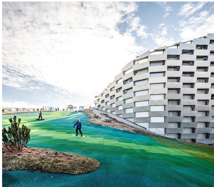
Figure 11. Copen Hill Building, Green Roof. (Dağtekin, 2020.)
