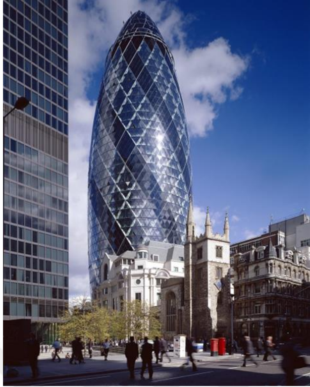
Figure 12. Swiss Re Building, London / England. (www.tricon.co.uk)
