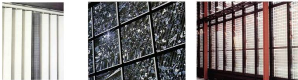
Figure 5. PV Panels Using as a Solar Control Element and Facade Cladding (Yilmaz, 2005)
