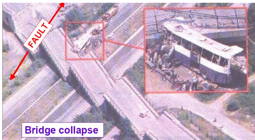
Figure 3.23 Reinforced Earth Ramp Walls and collapsed bridge, Arifiye
