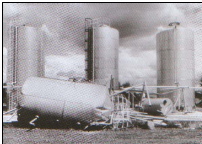
Figure 3.15 Overturned milk silo near Edgecumbe
