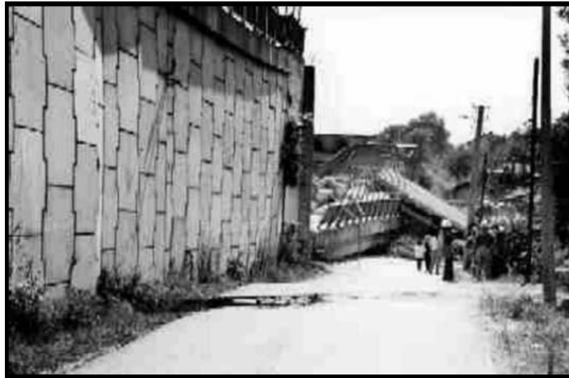
Figure 3.22 Arifiye Reinforced Earth ramp wall
