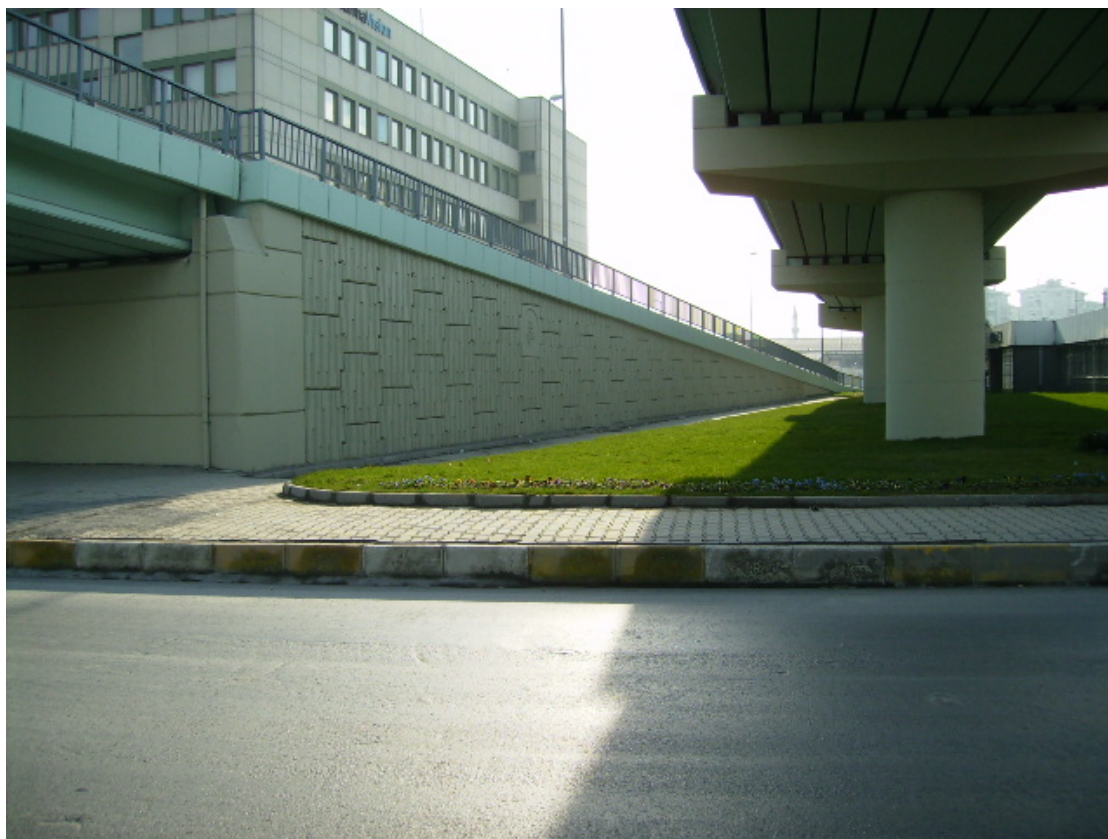
Figure 6.1 Davutpaşa Interchange Reinforced Earth Walls
