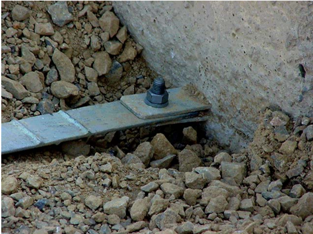
Figure 2.15 Connection Parts in Steel Strips
