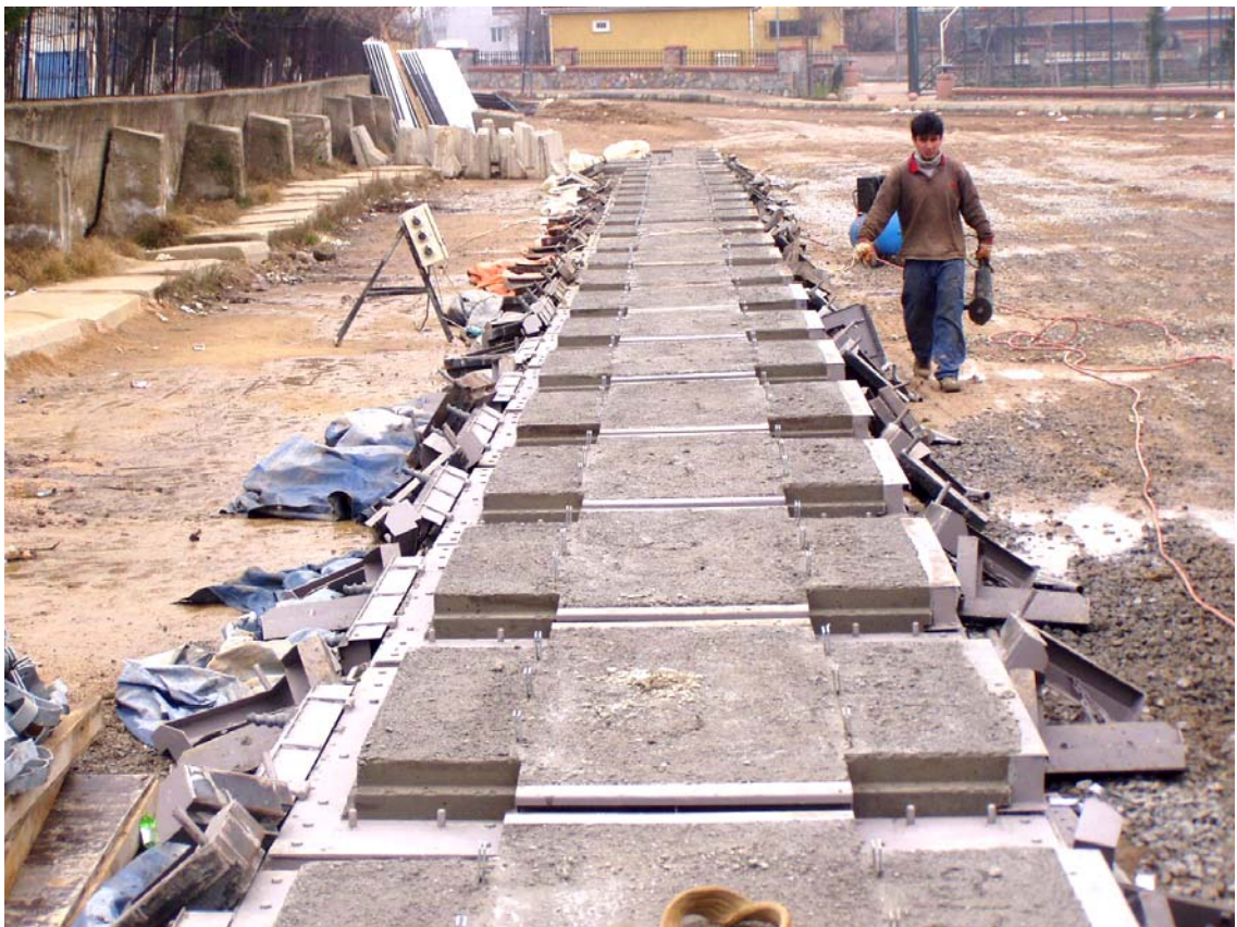
Figure 2.14 Reinforced Earth Panels
