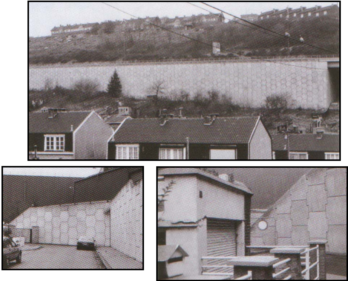
Figure 3.10 Views of one of the walls at Jemeppe and the neighboring garage
