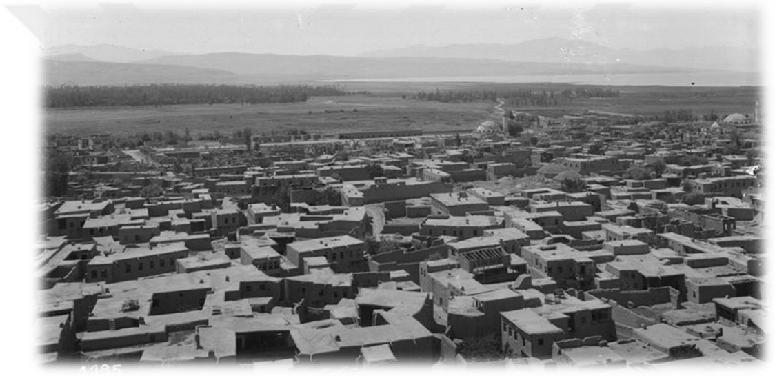
Fotoğraf-1: 1918 Öncesi Eski Van Şehri.( https://www.google.com.tr/search?q=eski+van+%C5%9Fehri&tbm=isch&source=iu&ictx=1&fir=5XY4njQKanaCIM%253A%252CPu9x3jV2XblnM%252C&usg=mvZffe4WkCqb4fNG7pKMxpzEjUY%3D&sa=X&ved=0ahUKEwi0yLj06bXcAhUCZVAKHSo-BU4Q9QEIMDAD#imgrc=5XY4njQKanaCIM ). (E.T: 22.07.2018).
