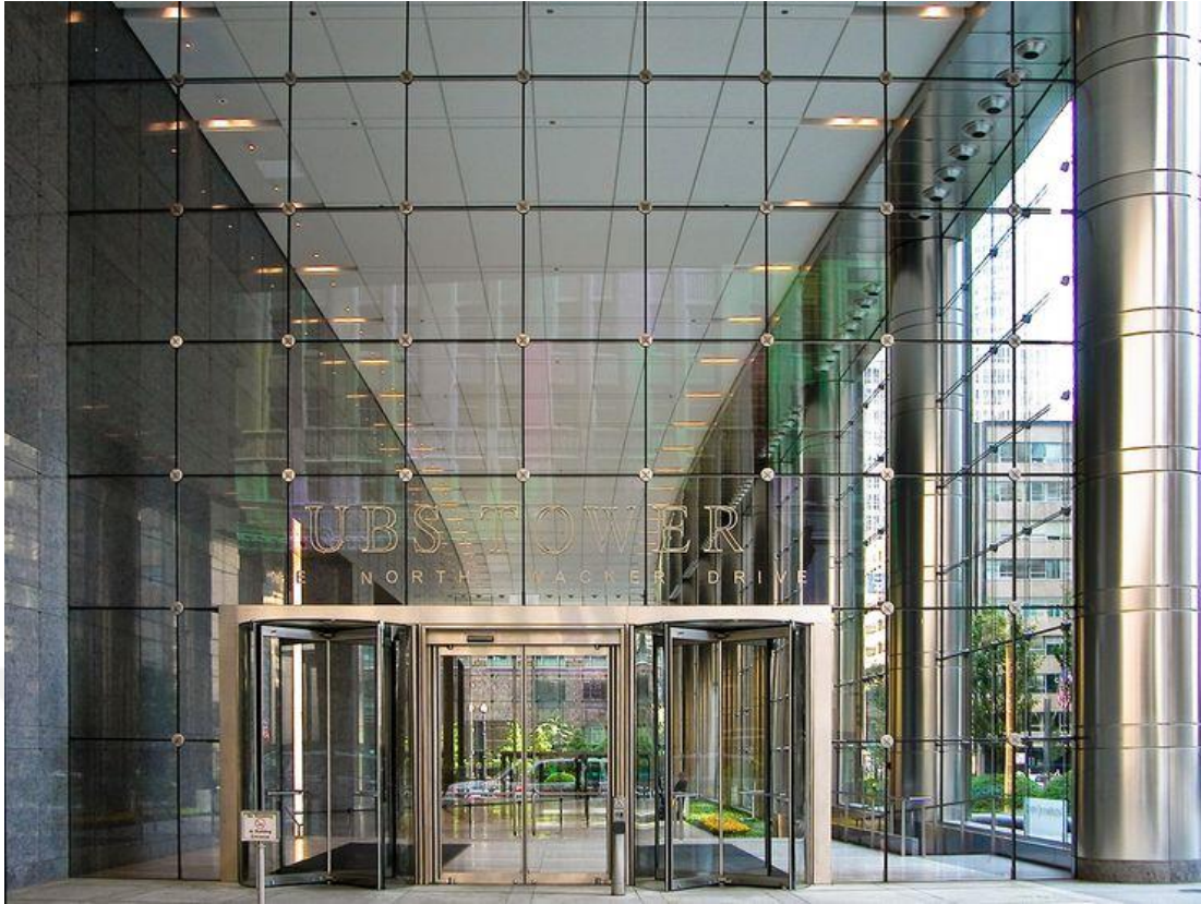
Figure 2.5 : Cable-net facade (Url-7).
