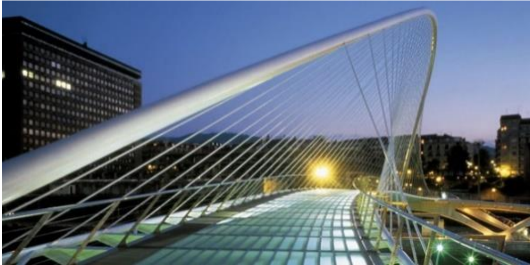
Figure 2.4 : Campo Volantin Bridge, 1997, Bilbao, Spain 1997 by Calatrava (Url-6).
