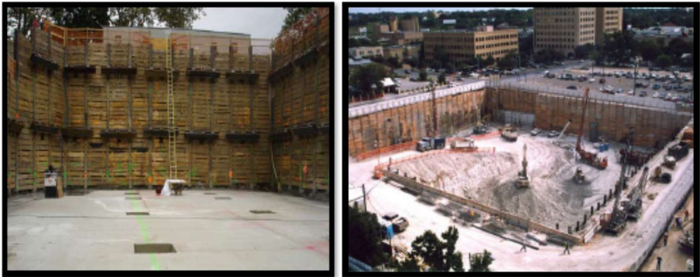
Figure 5.5 Soldier beam& lagging
