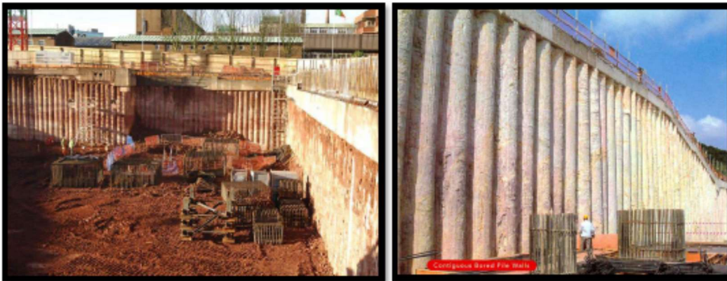
Figure 5.7 Bored pile walls
