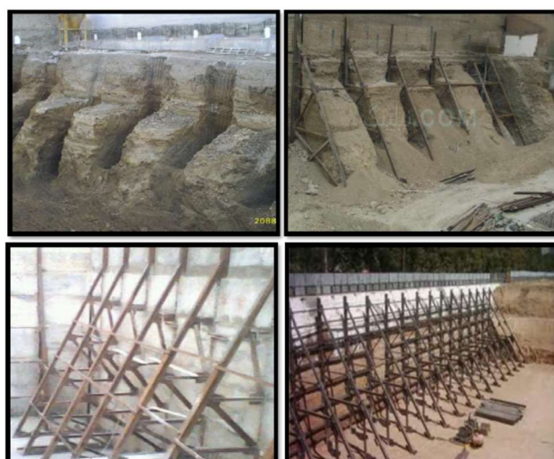
Figure 5.15 Truss-rocker implementation
