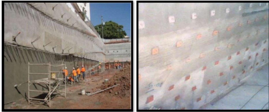
Figure 5.10: Soil nailing execution.
