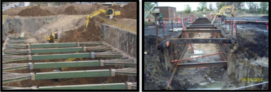
Figure 5.4: Braced Wall
