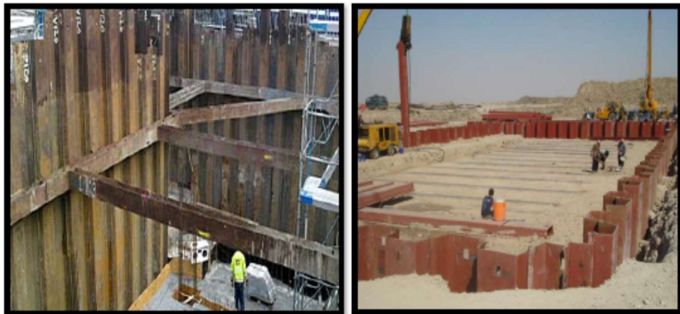
Figure 5.6 Braced sheet pile
