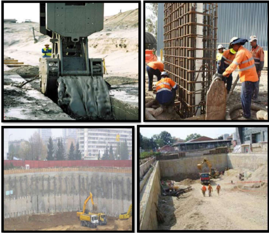
Figure 5.8 Diaphragm walls-Slurry wall
