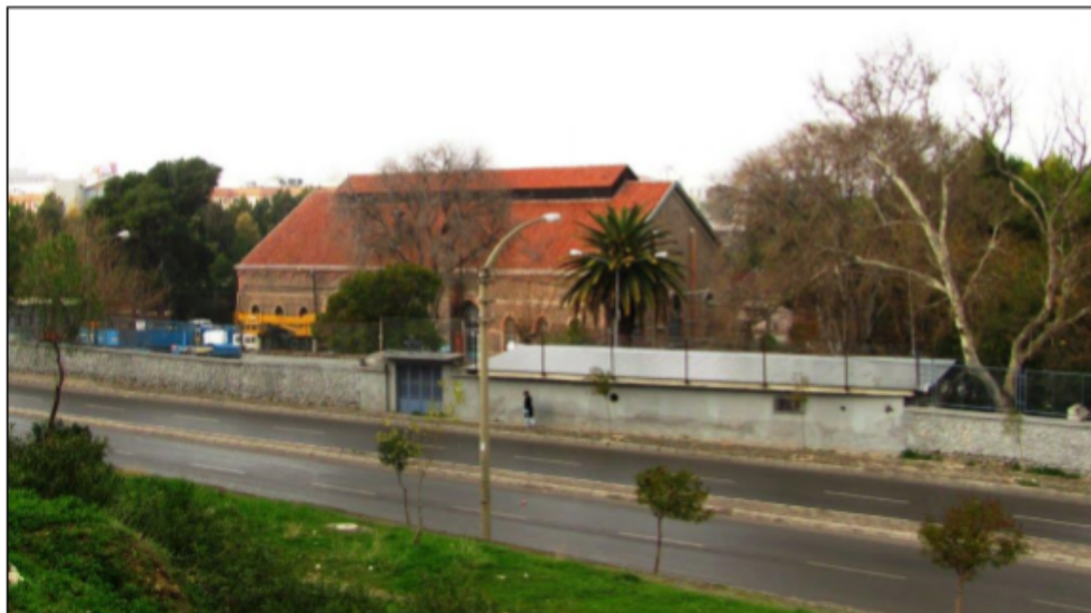
Figure 4.16. The water pumping station providing potable water for the city from 1897 to 1988 (Source: Aksoy S. 96)
