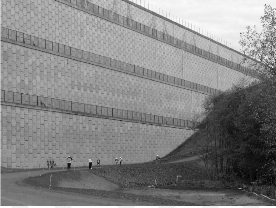
Şekil 2.9 : Sea-Tac Havaalanı, WA (Reinforced Earth Company, ABD).
