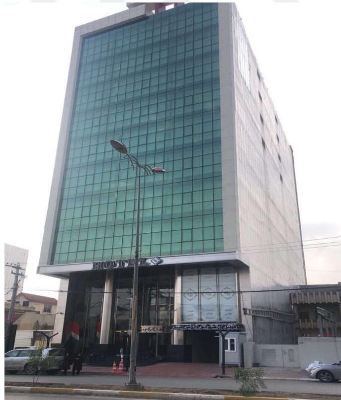
Figure 4.21 Shows presence of heavy overhang
