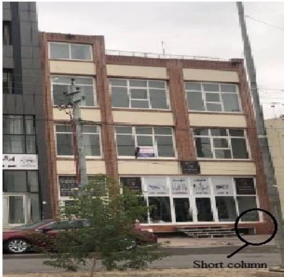
Figure 4.24 Presence of short column in Brayaty Quarter in Erbil City
