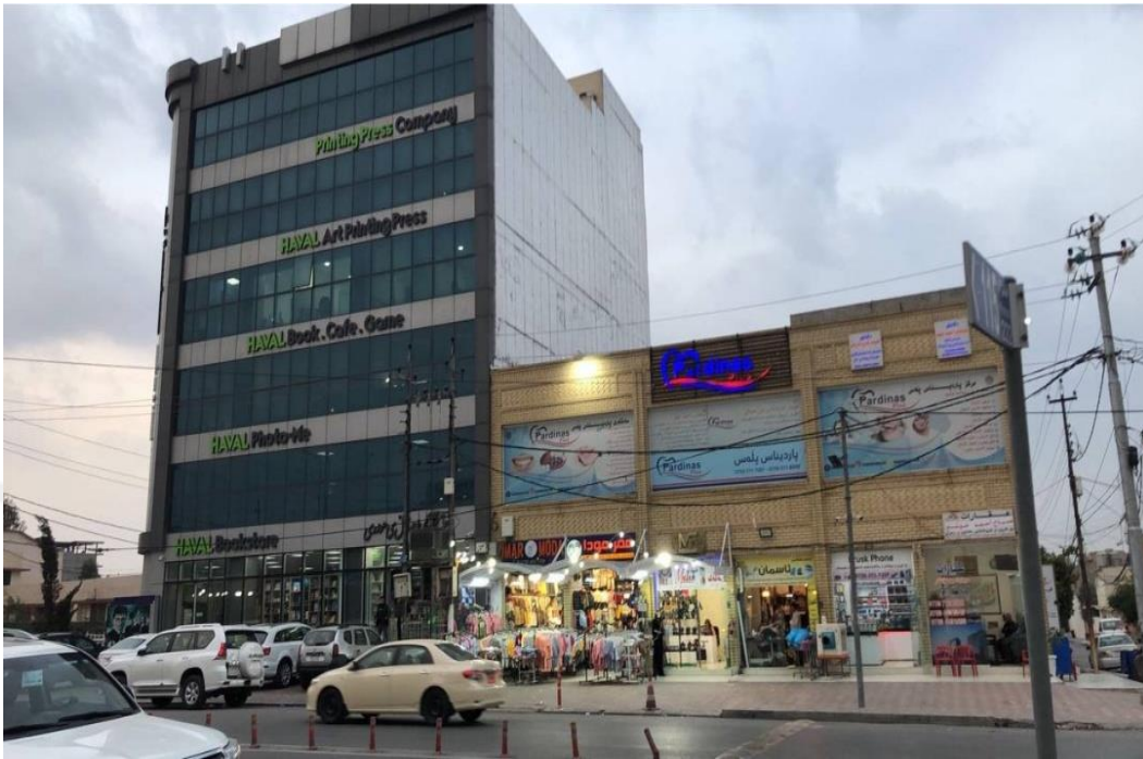
Figure 4.26 Pounding one building is two or more stories taller than the other
