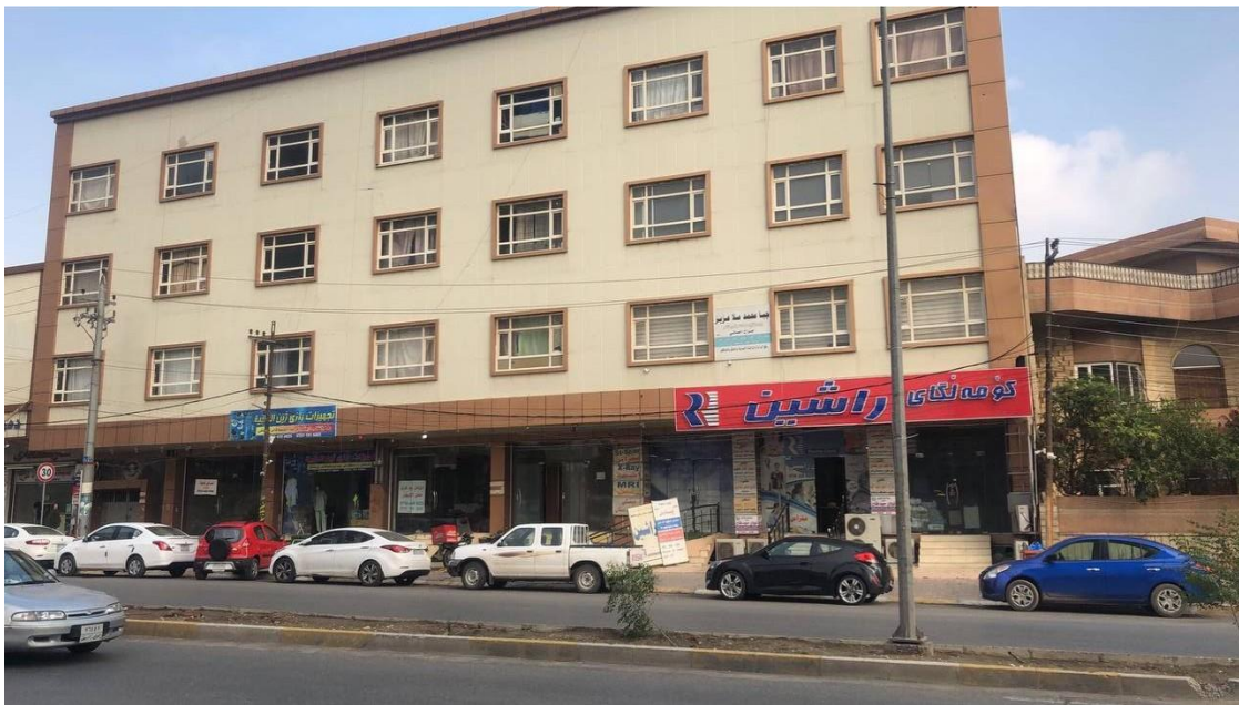
Figure 4.4 Four storey building example in Brayaty Quarter in Erbil City
