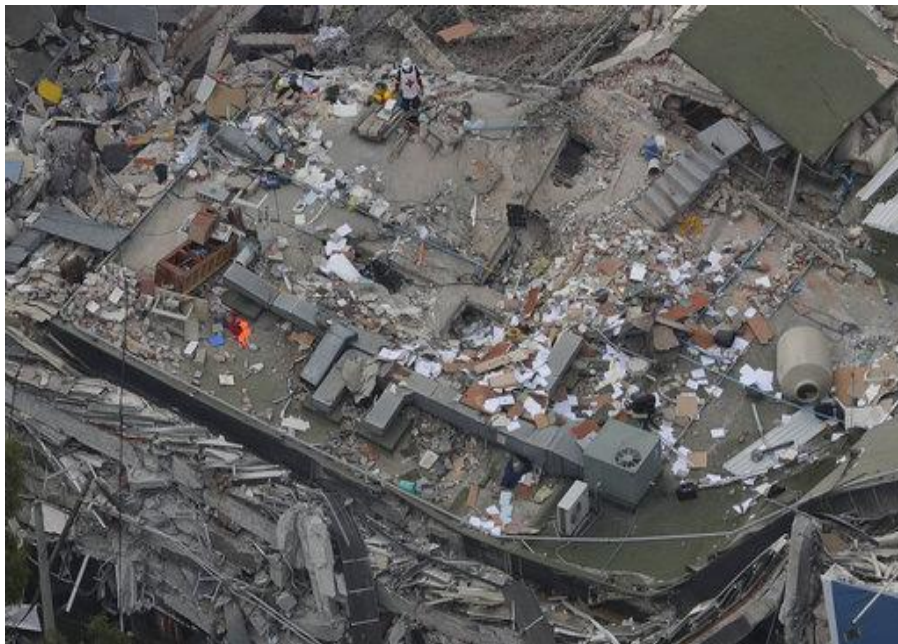
Figure 2.10 Soft soil makes Mexico City shake like it was built on jelly
