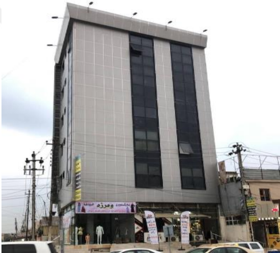
Figure 4.25 Pounding end building
