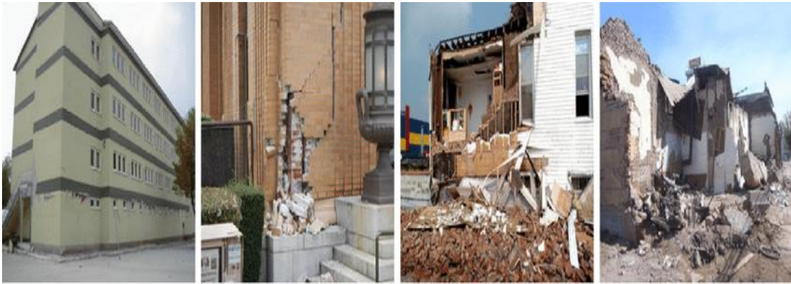
Slight-damage (0.25) Moderate-damage (0.5) Heavy-damage (0.75) Total-destruction (1)
