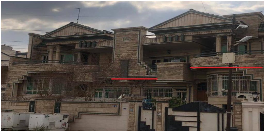
Figure 4.12 The two red lines illustrate split level in a building in Brayaty Quarter in Erbil City
