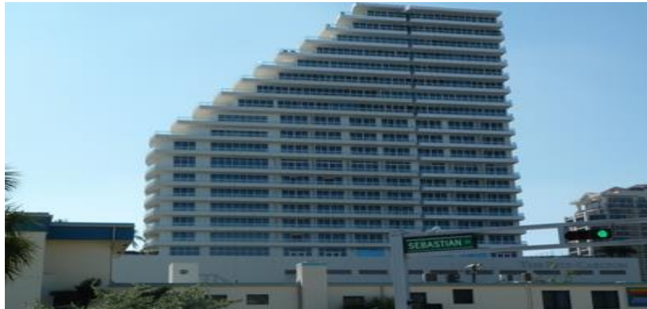
Figure 2.6 Vertical irregularity
