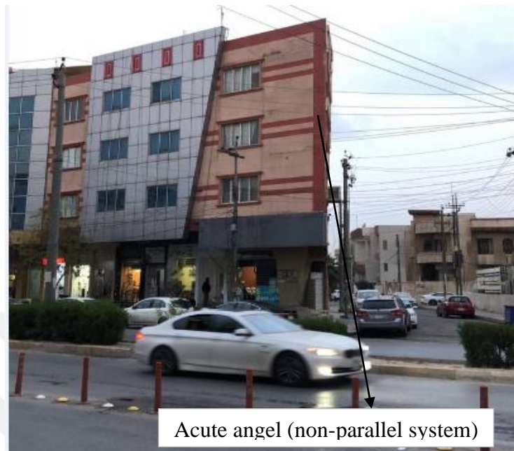
Figure 4.15 The front of the building and the side on the right do not form 90-degree angles in Brayaty Quarter in Erbil City
