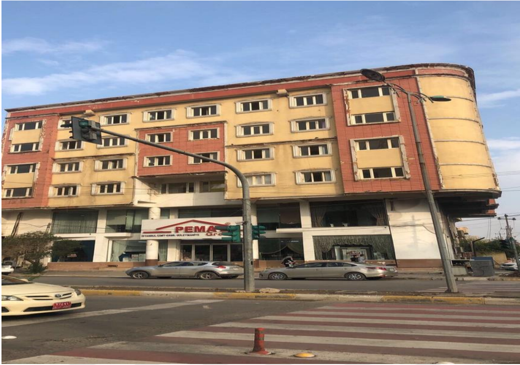
Figure 3.5 Sample of reinforced concrete building in Brayaty Quarter, solving by (Sucoğlu and Yazgan, 2003) method
