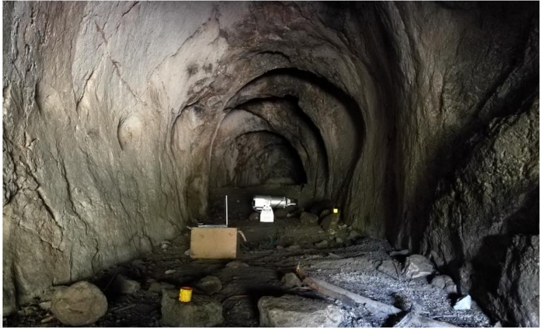
Figure 21 The unfinished tunnel in Büyükkaya (Repola, 2020)
