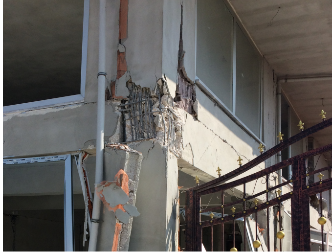
Figure 1.2 Joint failure in a building built in mid-2000s from Samandağ, Hatay [4]
