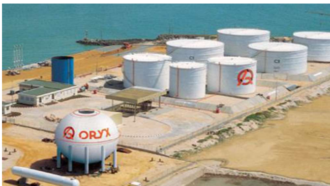
a- Installation at ORYX terminal.
