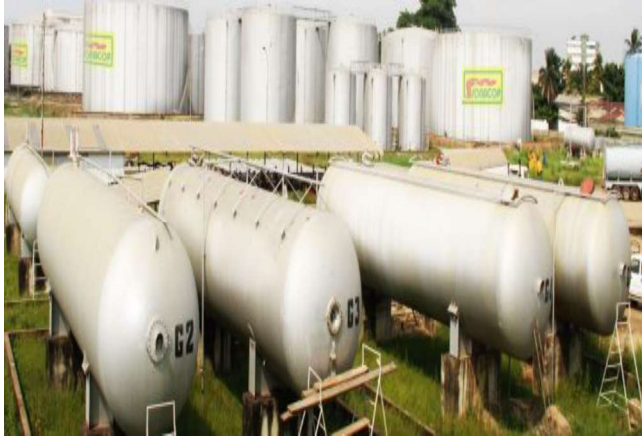
b- SONACOP connection installation.
