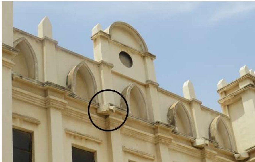
Figure 71. Indararo/ roof gutters in Gombe palace (Author's Archive, 2023).
