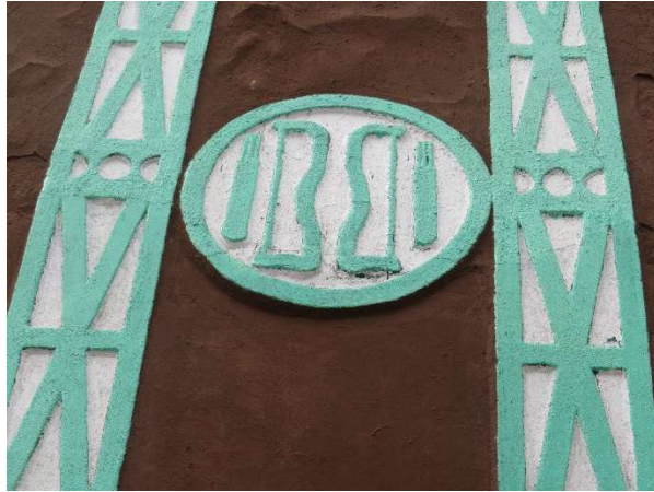
Figure 45. Bow and arrow ornament in the Bauchi Palace (Author's Archive, 2023).
