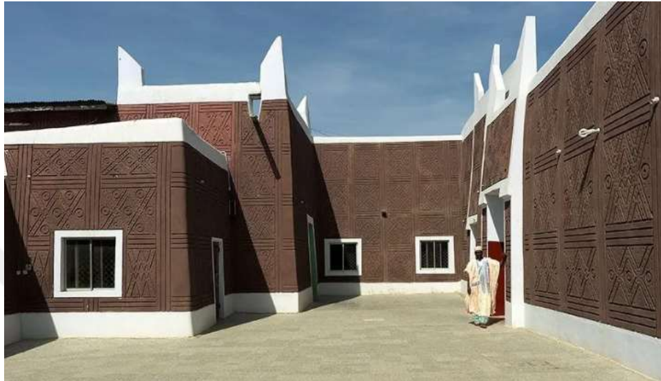
Figure 35. A section from the Kano palace (Samuel, 2022).
