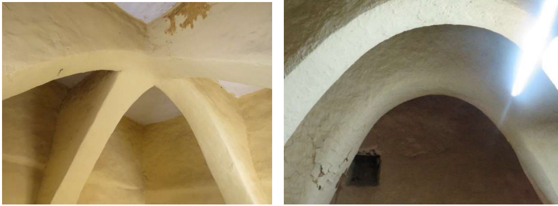
Figure 48& 49. Ribbed vault and arch structural members in the palace (Author's Archive, 2023).
