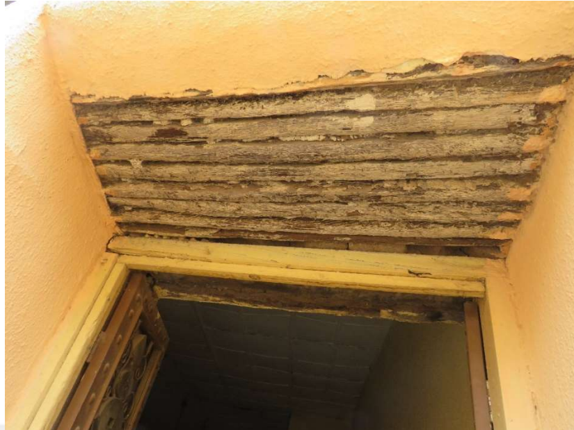
Figure 27. Azara timber used for roofing (Author's archive, 2023).
