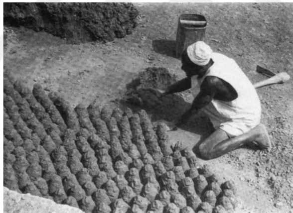
Figure 31. Making of tubali mud bricks
