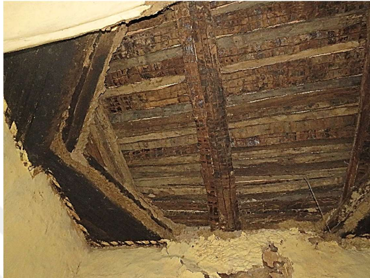
Figure 41. Exposed timber used in the construction of the palace (Author's Archive, 2023).
