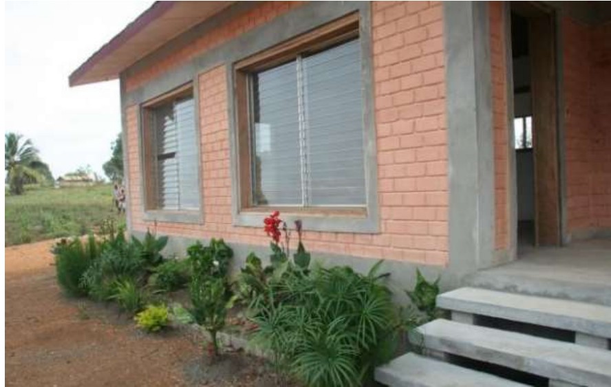
Figure 79. Adobe bricks in a house in Liberia (Gbatu & Li, 2019).
