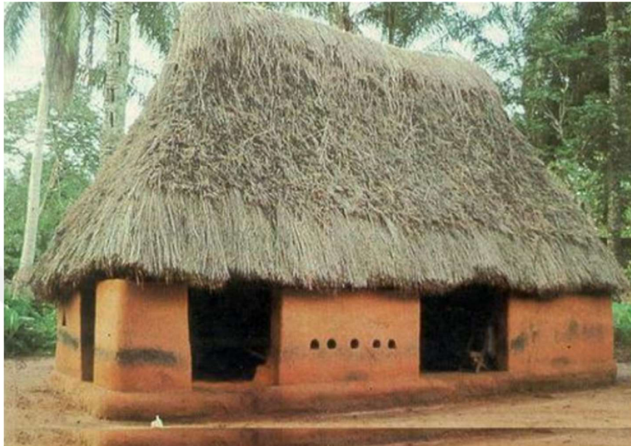
Figure 19. A steeply pitched roof from Igbo vernacular architecture (Kabir, 2016).
