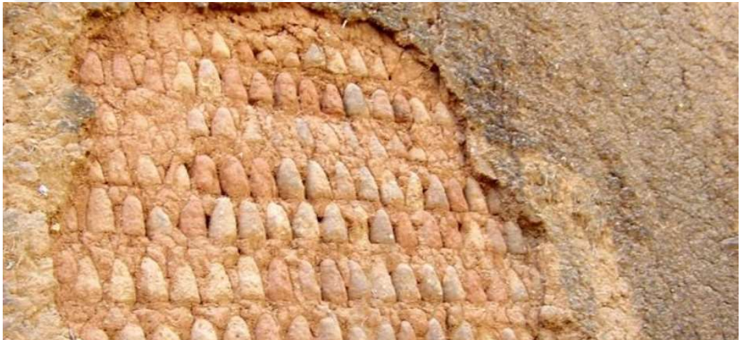
Figure 26. Mud bricks or tubali used in wall construction (Kabir, 2016).
