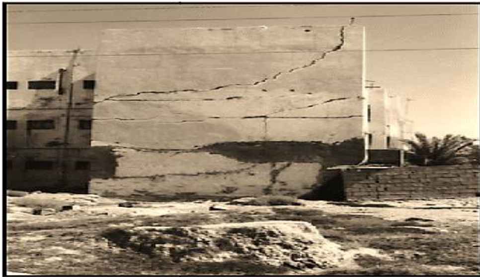
Plate 2.2 Collapse of a building in Al-Anbar University in Al-Ramdi City [59]
