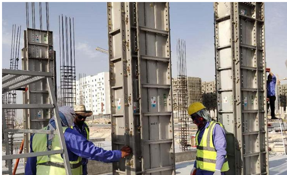
Figure 16 Assembly of aluminium column formwork
