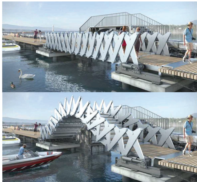
Figure 2.6. Jet d'Eau movable footbridge (Source: Bouleau and Guscetti 2016)
