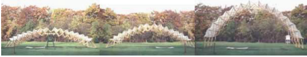
Figure 2.3. Transformation sequence of Cable-scissor arch (Source: Kokawa 1997)
