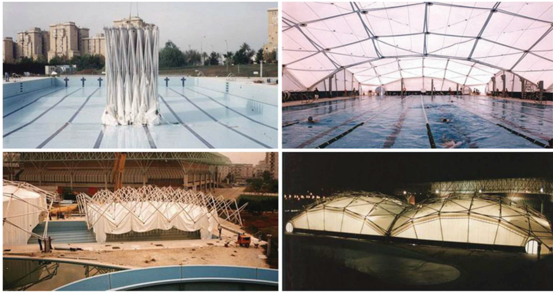
Figure 2.17. Deployable roof structure composed of SLEs in Seville (Source: Escrig and Sánchez 2006)
