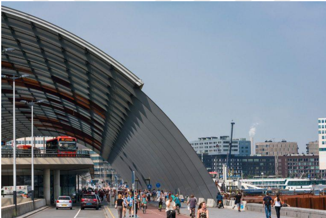
Figure 5.7 : Relation between slow traffic passage and the bus terminal (Bentham Crouwel Architects).
