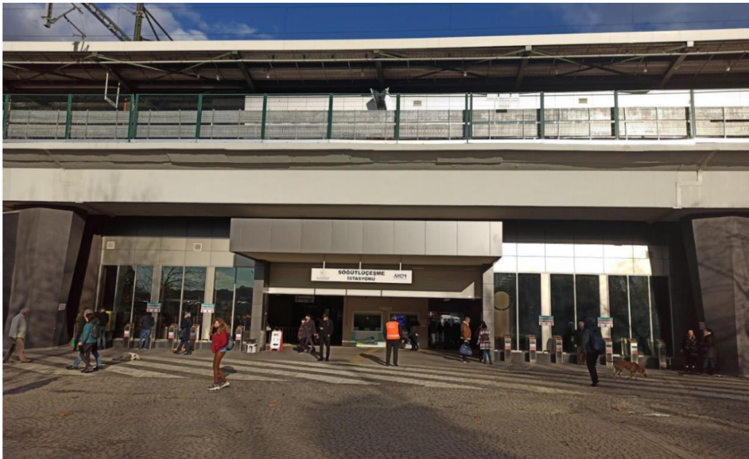
Figure 6.13 : Marmaray Sogutlucemesme Station south entrance.
