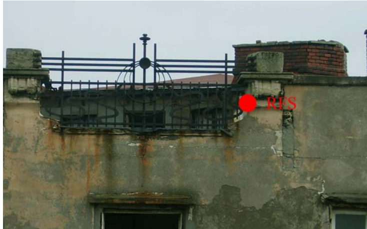
Figure 21. Figure showing the place of Roof Floor Sample (RFS) taken from.
