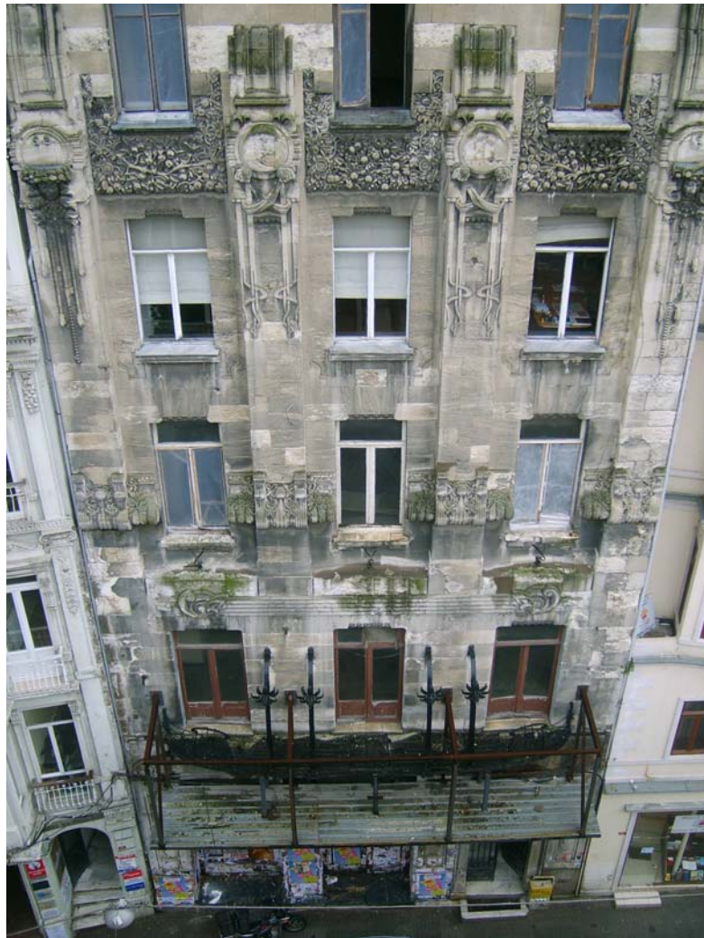
Figure 32. Present condition of the Botter Apartment
