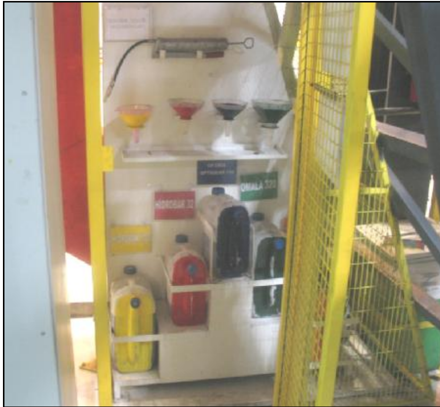
Figure 4.14. Lubrication Station of Komatsu Line
