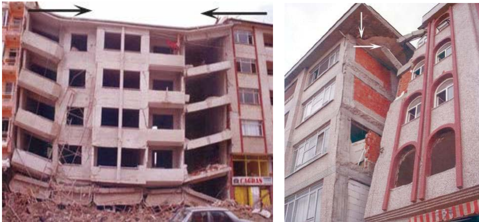
Figure 3.31. Pounding due to the torsion between adjacent buildings (Source: İstanbul Büyükşehir Belediyesi Devlet Arsivi, 1999)
