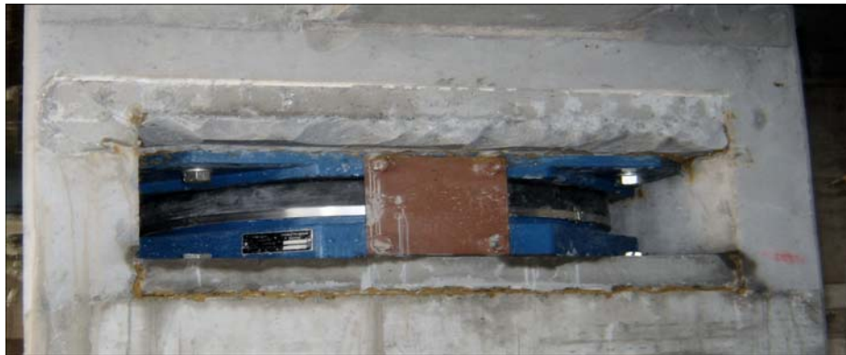
Figure 6.18. Replacement of FPS isolators to columns for retrofit project
