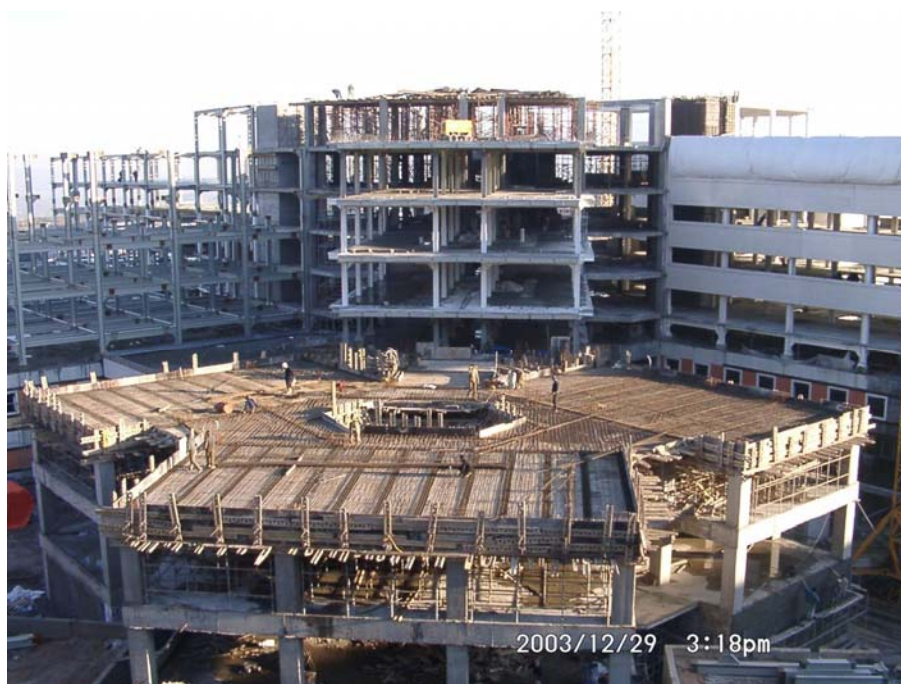
Figure 6.9. Construction stages of Kocaeli Hospital
