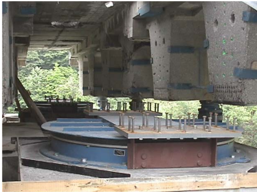
Figure 6.27. Locations of FPS isolators at bolu Viaducts
