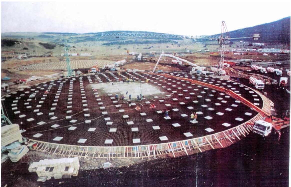
Figure 6.11. Locations of isolation devices for LNG tanks
