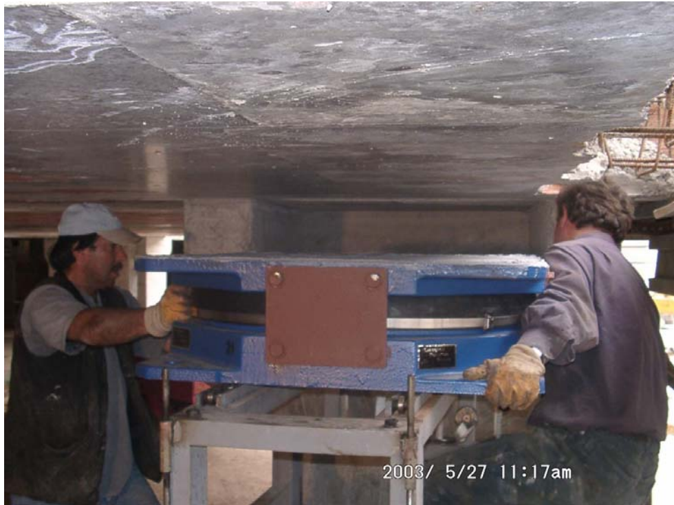
Figure 6.18. Replacement of FPS isolators to columns for retrofit project
