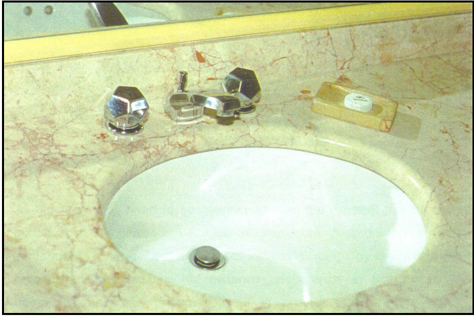
Figure 4.9. The faucet fittings and marble claddings in typical standard room of Hotel A before refurbishment. (Source: Ozgurel, 2001: 92).
