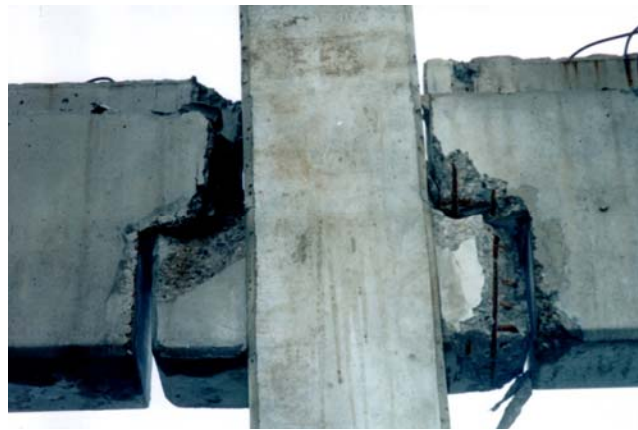
Figure 1.3. An example of common type beam-column connection [9]
