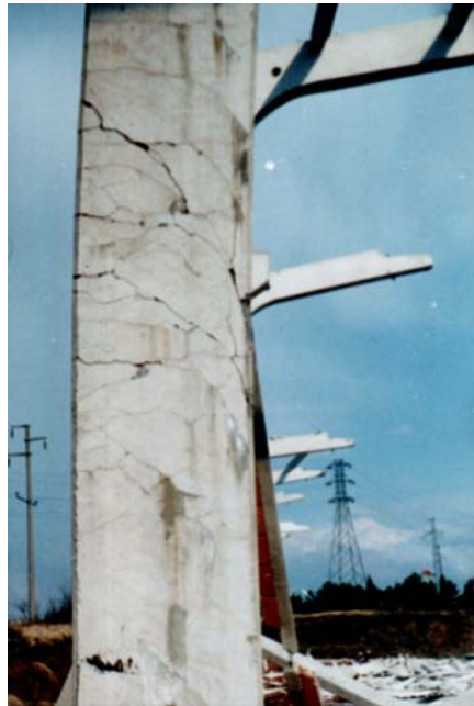
Figure 1.2. Flexural column failure at the \frac{1}{3} rd column height [9]
