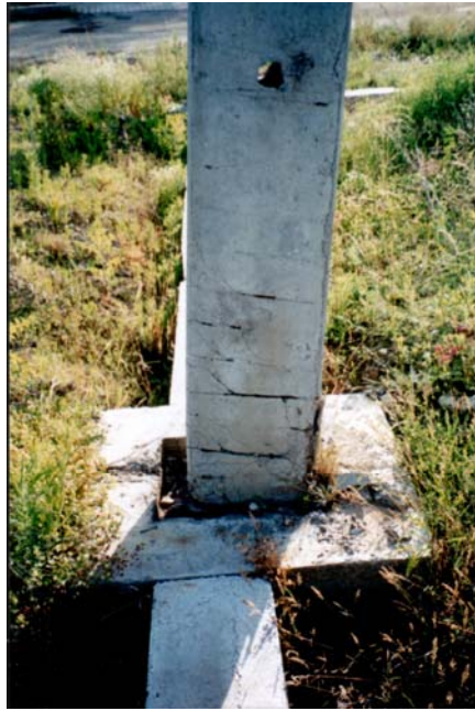
Figure 1.1. Flexural column failure at the base [9]
