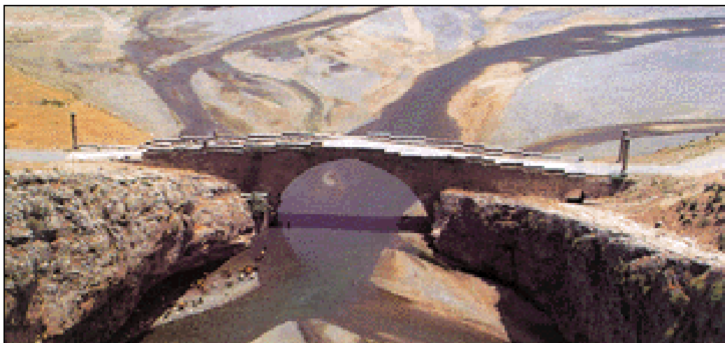
Figure 2.8. Cendere Bridge, Turkey [26]
