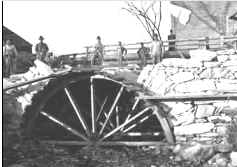
Figure 2.4. A typical view of centering [13]
