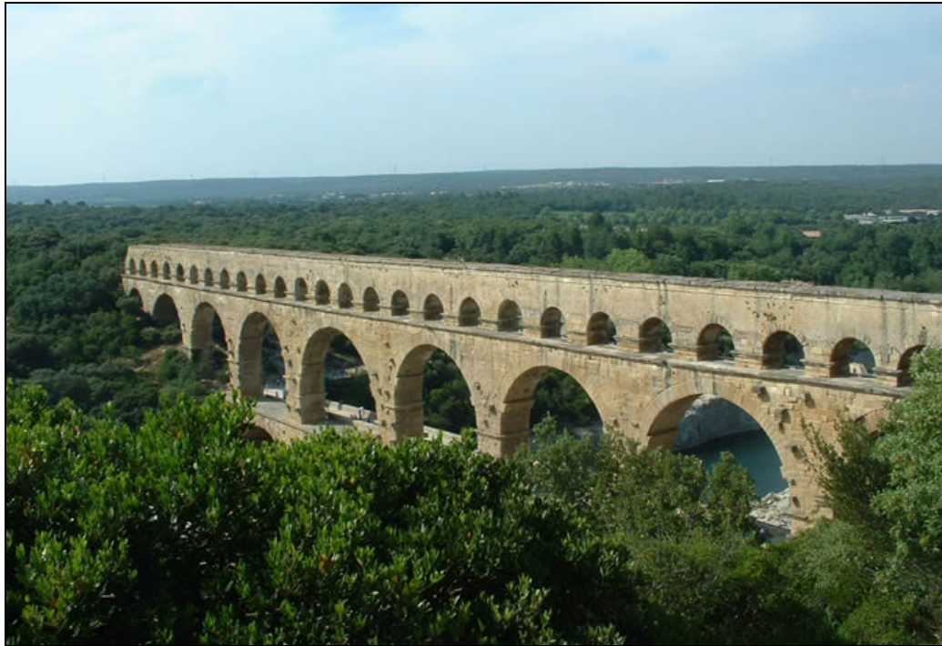
Figure 2.7. Pont du Gard, France [2]
