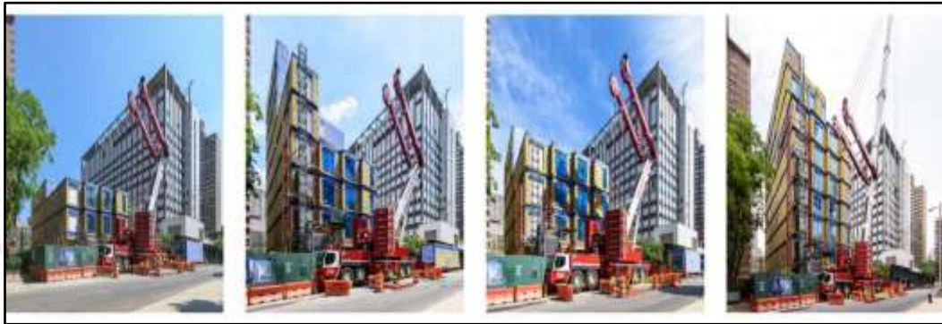
Figure 2.10: Stacking of the Modular Units (LILAC, 2019).
