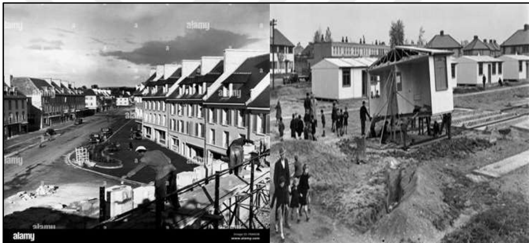
Figure 2.3: Assembly of Prefabricated Housing Units In Post-War Germany to Accelerate Construction Timelines (Diefendorf, 1993b).
