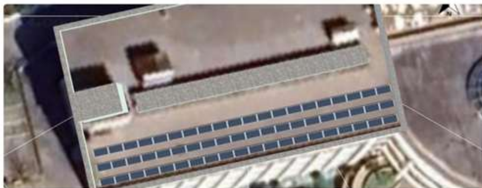
Figure 4.9. Completely covered roof with solar panels facing west.
