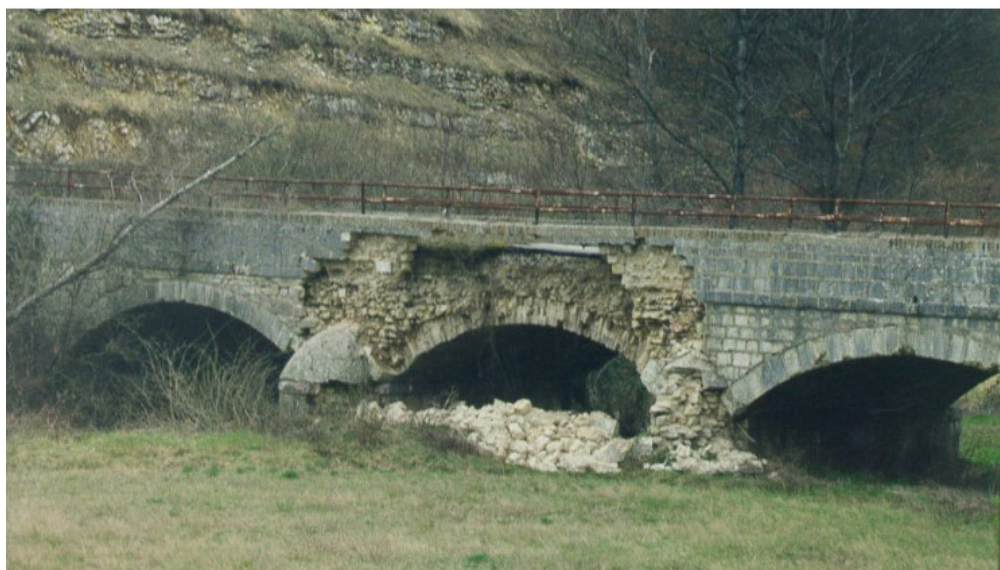
Figure 3.6 Collapse of spandrel of a masonry bridge during the Umbria-Marche earthquake of 1997
