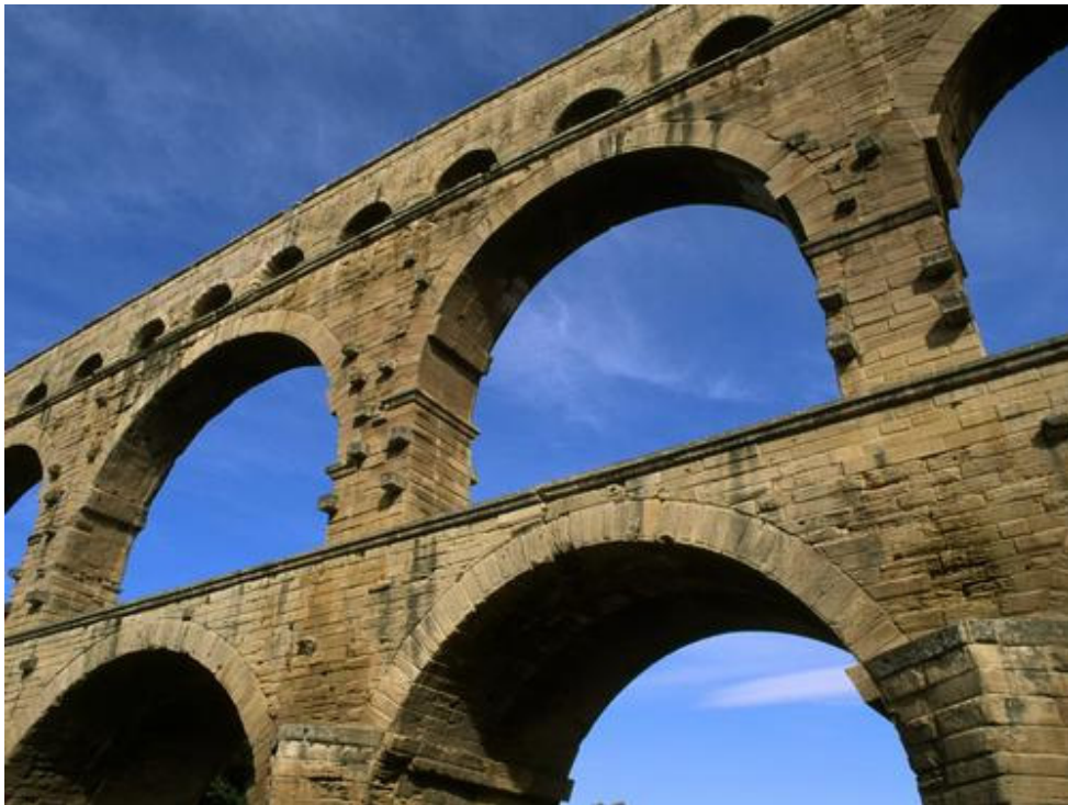
Figure 2.21 The Roman aqueducts in Nimes, France
